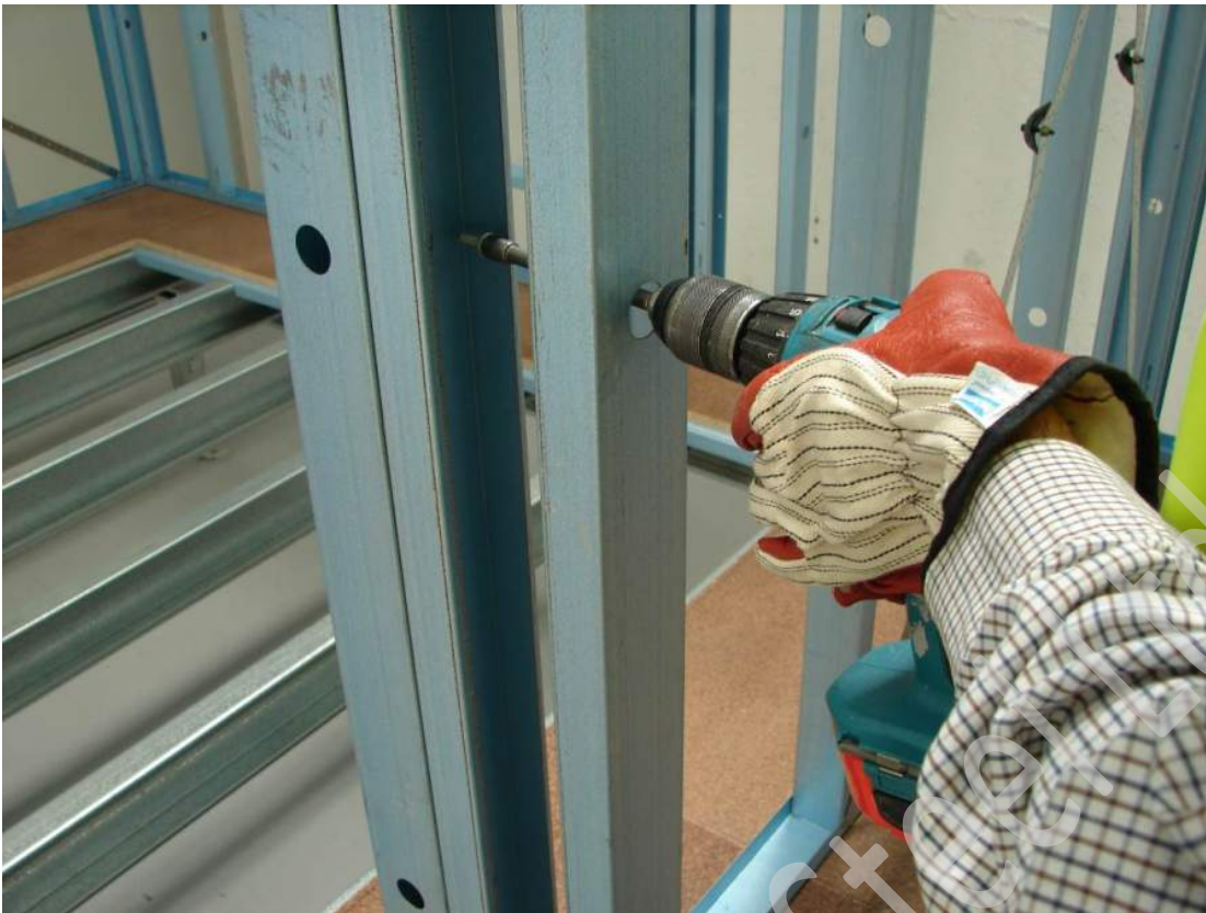
Figure 7.18 Position and fix final wall using extension bit.
