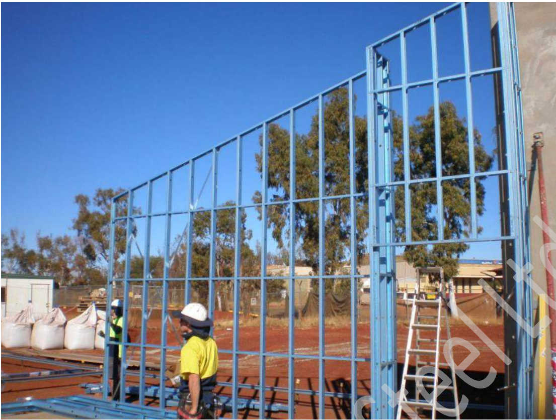
Figure 7.5 Place second wall in position using chalk line as a manual and flush against first wall.
