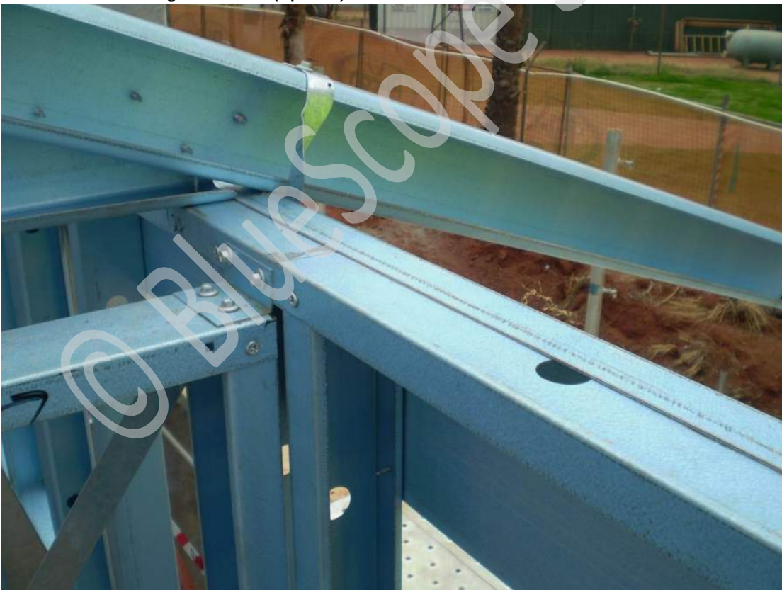
Figure 7.36 Internal to external fixing connections (Option 2)
