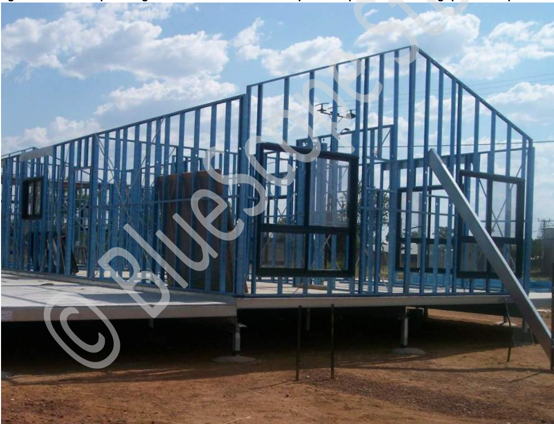
Figure 7.29 Wall up, plumbed, squared and fixed - ready to fit roof trusses
