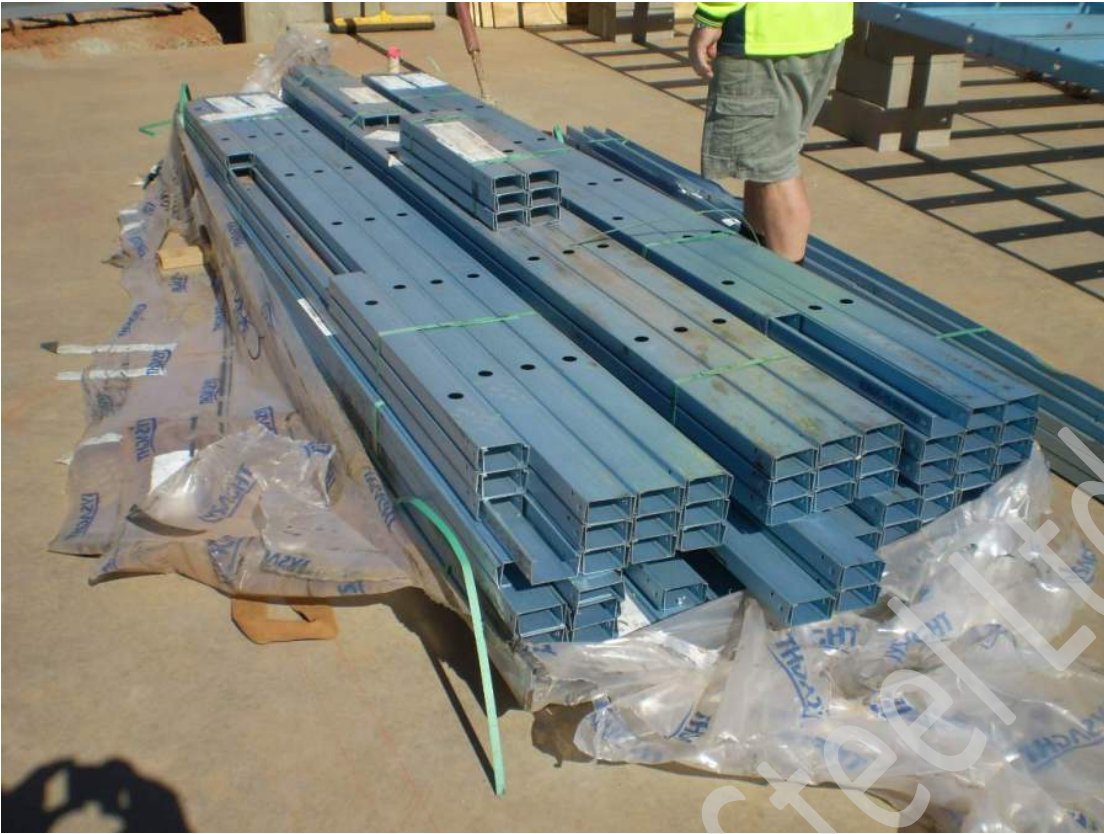
Wall frames are individually strapped & stacked in "stud" bundles, labelled with bundle numbers
