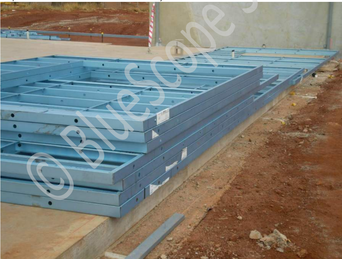
Stack wall frames in bundles close to the final installation position.
