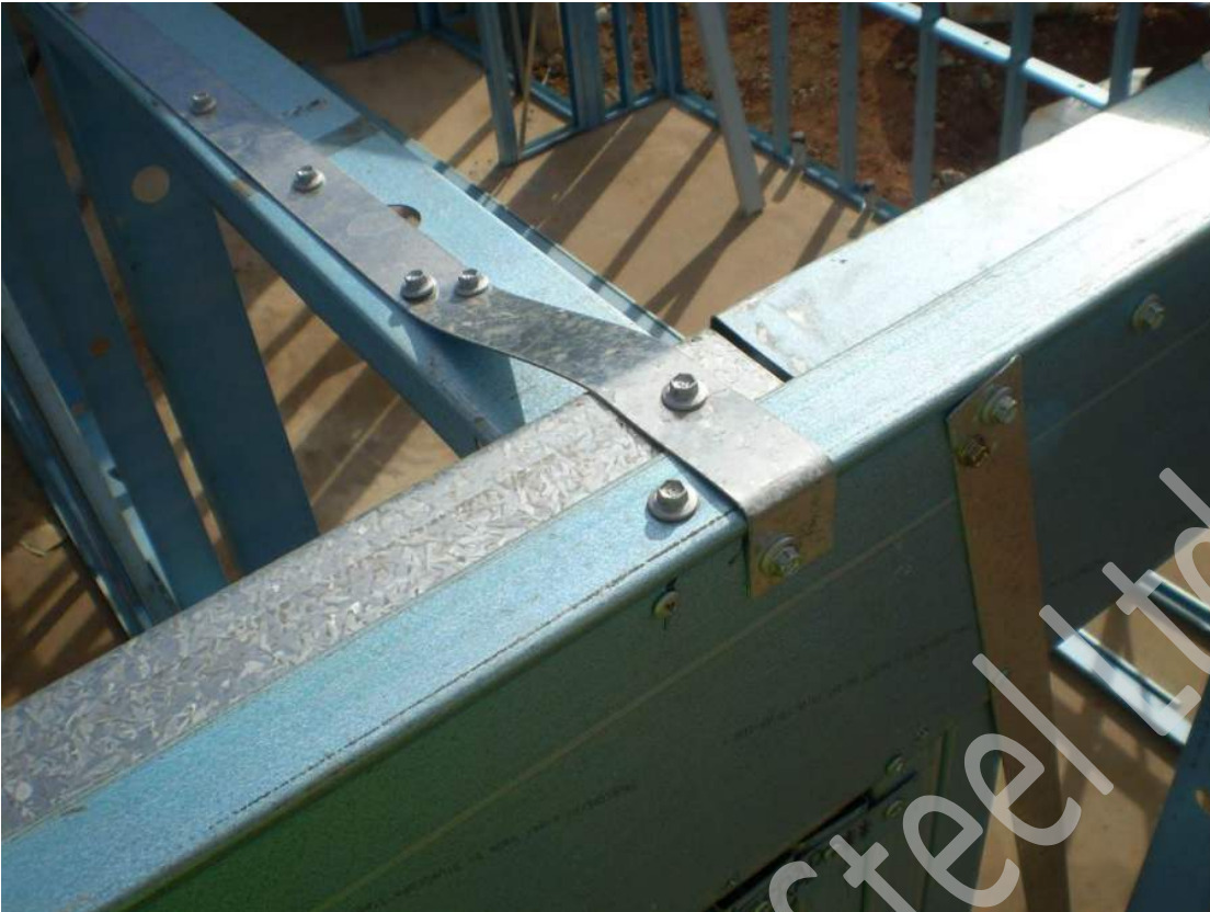
Figure 7.35 Internal to external fixing connections (Option 1)
