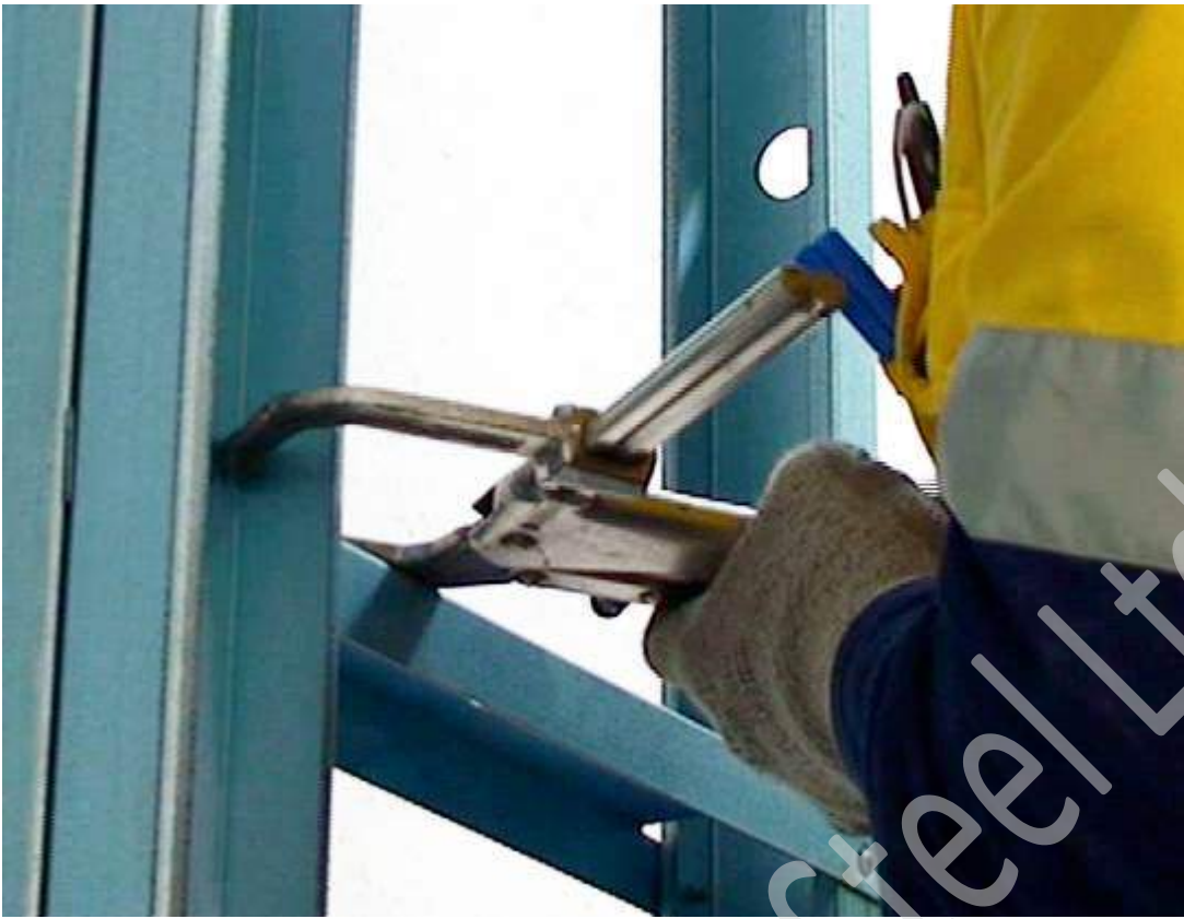
Figure 7.12 Use clamp to hold temporarily in position.
