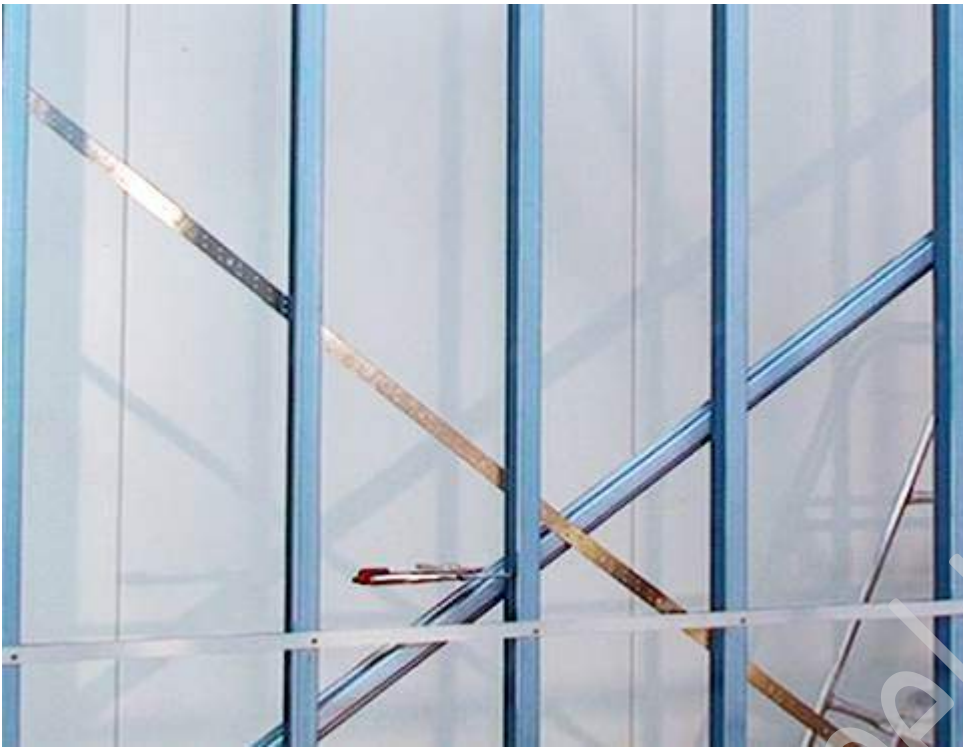
Figure 7.28 Use strap bracing and tensioner to set frame square and plumb. Note vice grips at mid-span.
