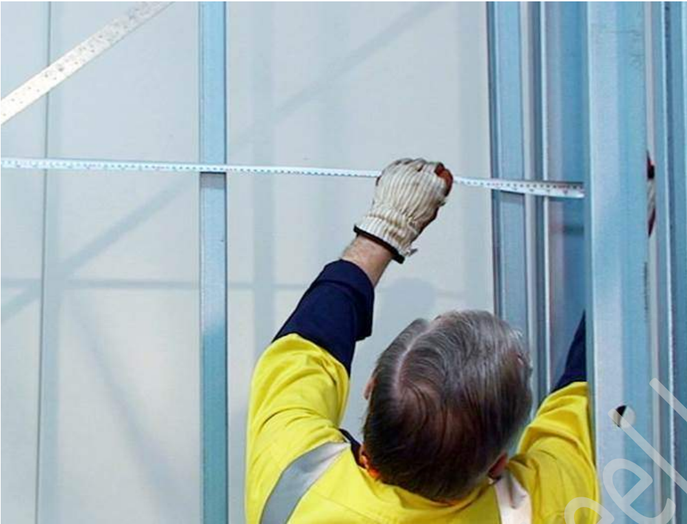
Figure 7.22 Measure lengths at bottom and top of wall to check frame is square.
