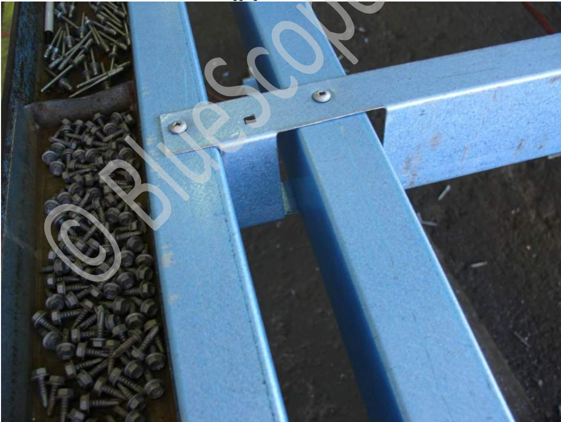
Nogging installation.
