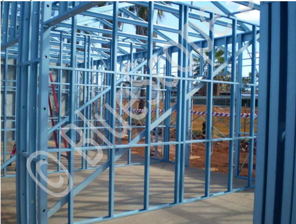
Figure 7.15 Position final wall.
