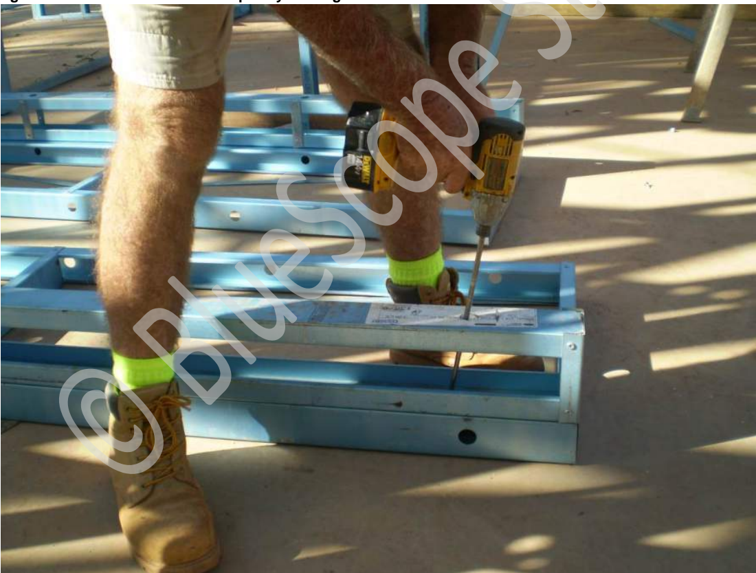
Figure 7.17 Join walls at corner using extension bit.
