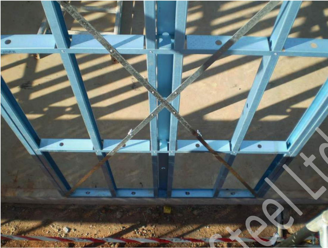
Figure 7.24 Check plumb and square and adjust as required.
