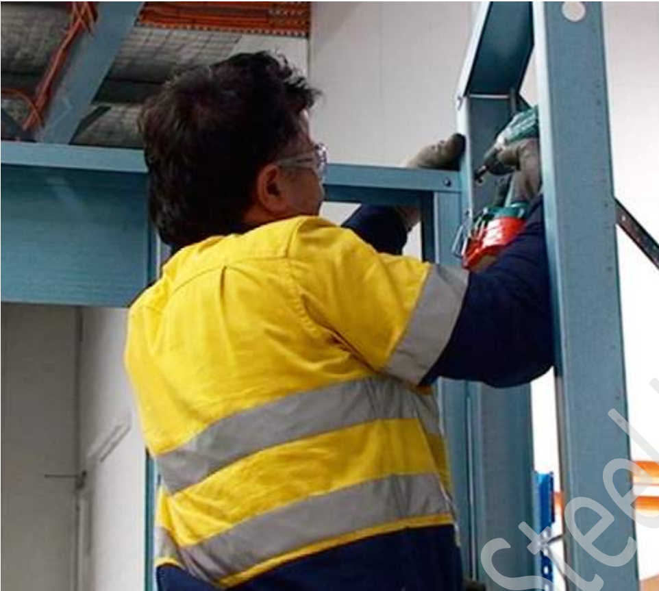
Figure 7.27 Once the frame is plumb and square, fix at the top of the wall.
