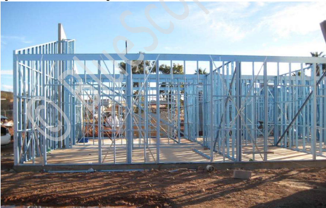
Figure 7.11 Interior walls are fixed into position.
