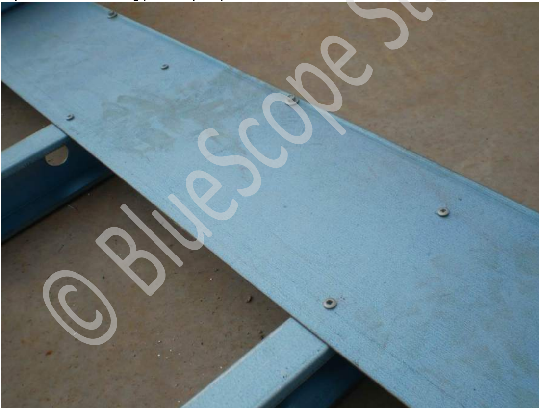
FIGURE 6.15- Tie-Down into suspended frame floor systems
