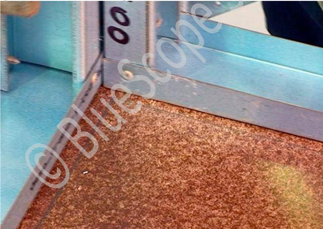
Figure 7.19 Align walls with chalk marks and put into final position before fixing.
