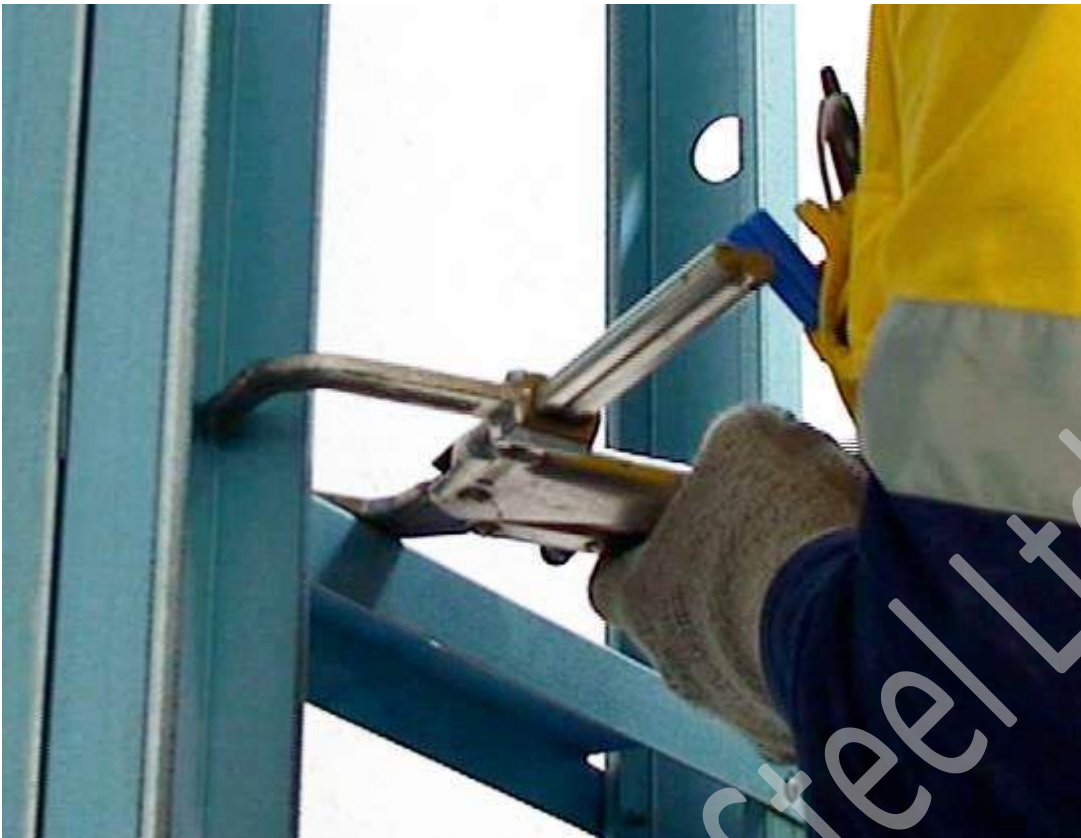
Figure 7.12 Use clamp to hold temporarily in position.
