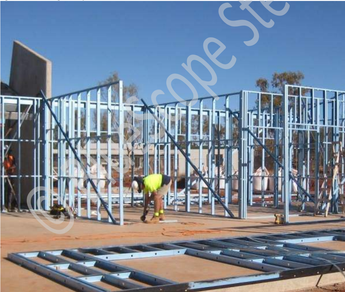
Figure 7.8 Affix temporary bracing as required.
