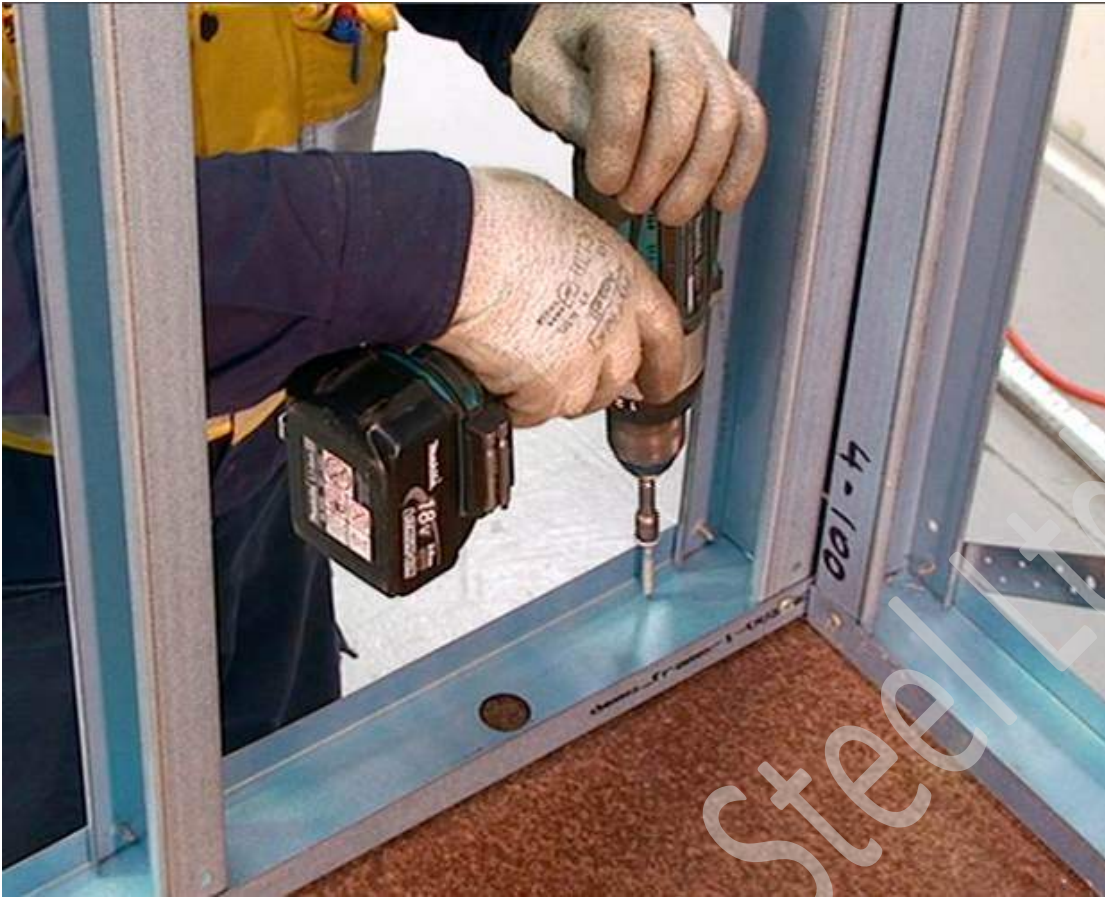
Figure 7.20 Screw bottom plate into final position on floor.
