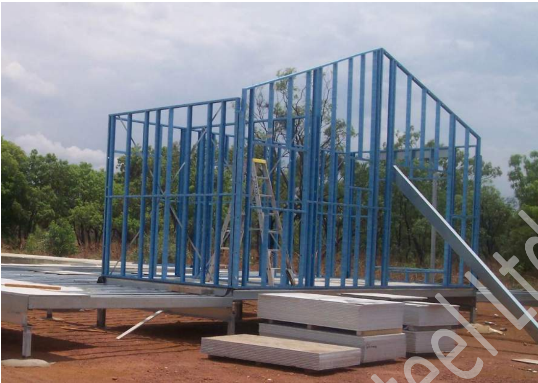
Figure 7.9 Structure with temporary bracing.
