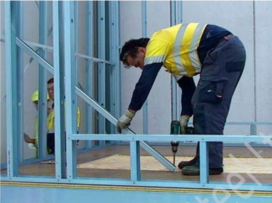
Figure 7.16 Remove last of the temporary bracing.
