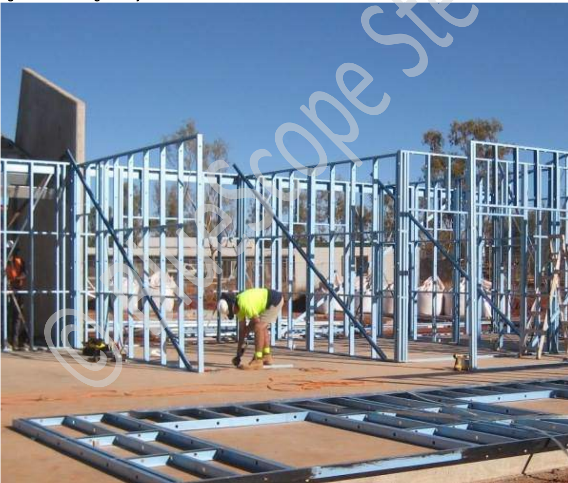
Figure 7.8 Affix temporary bracing as required.
