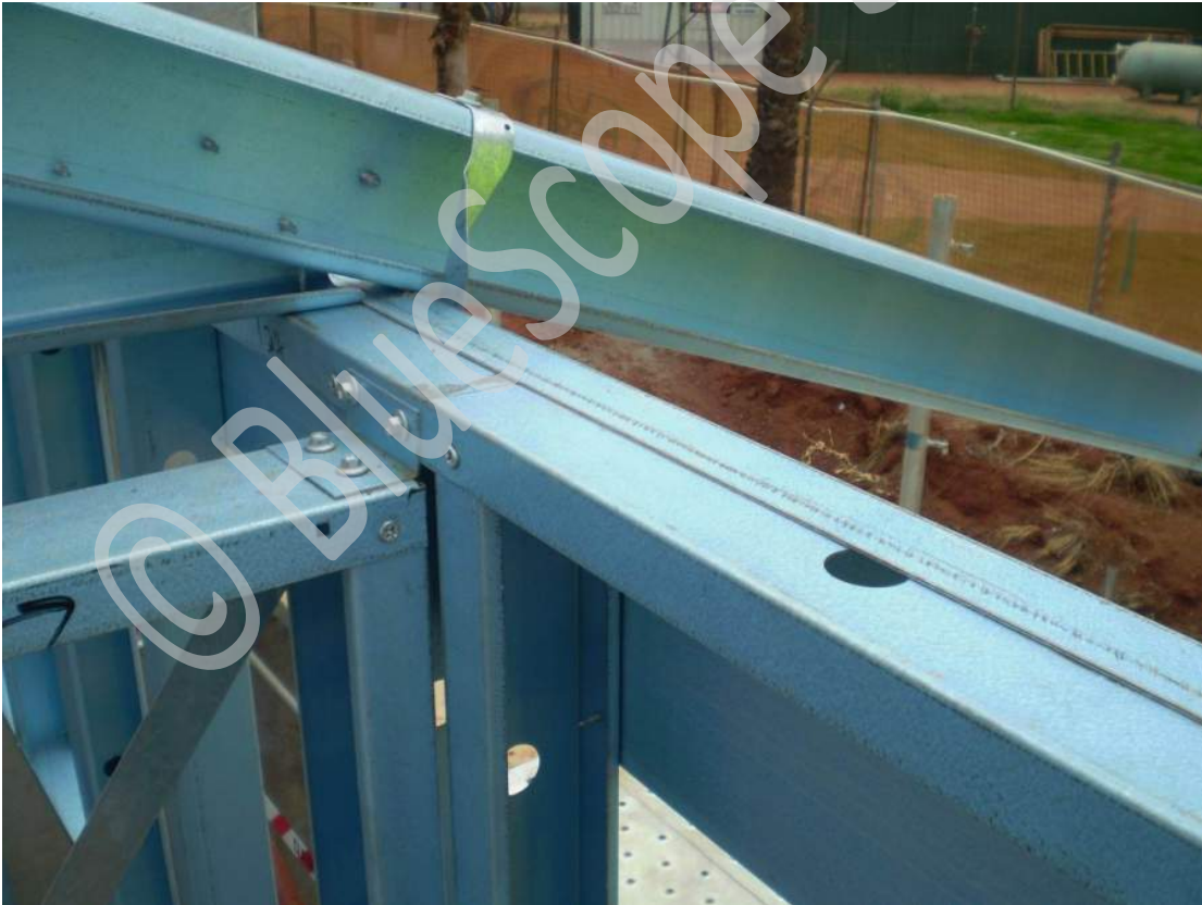
Figure 7.36 Internal to external fixing connections (Option 2)
