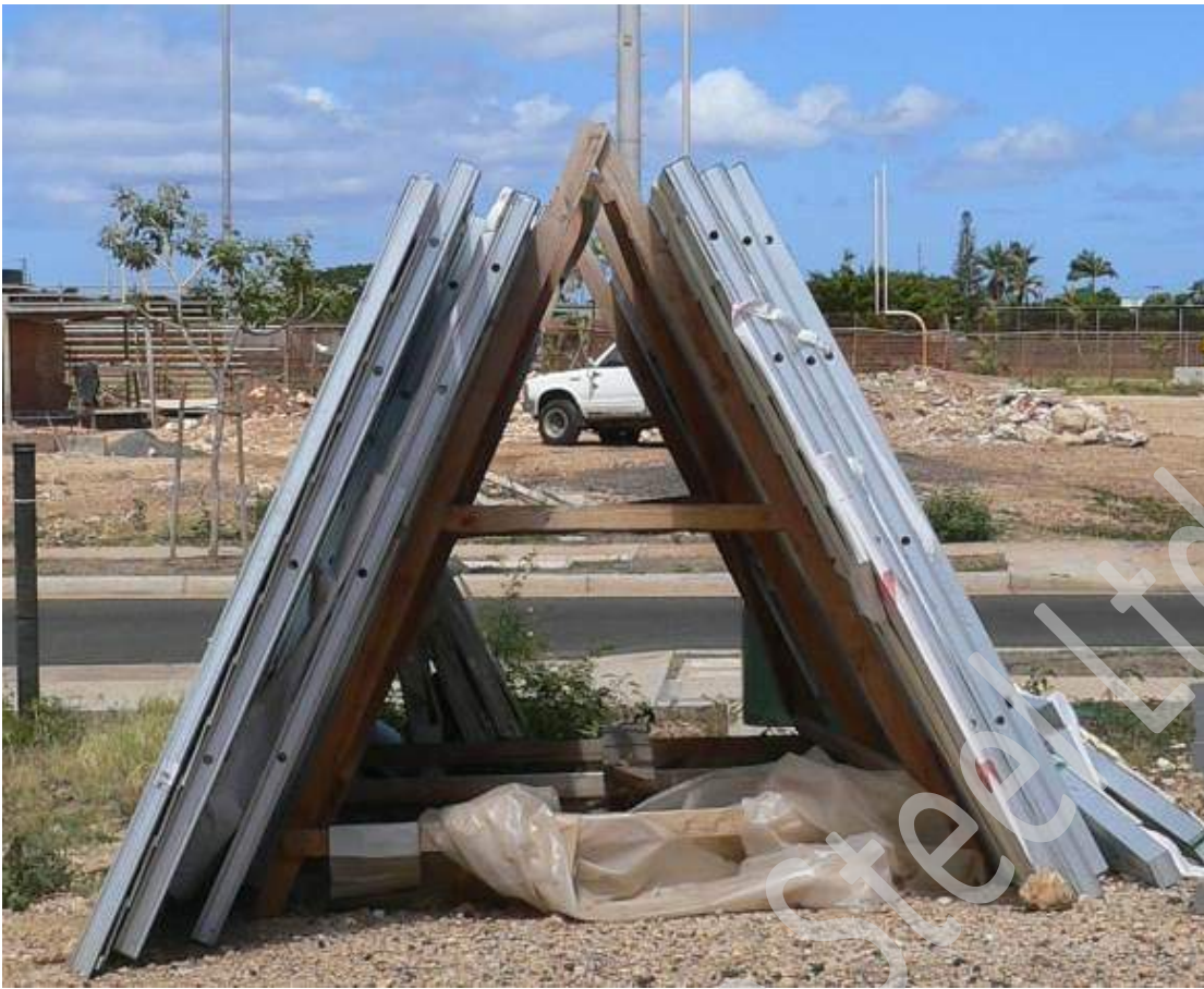
Figure 2.2.1 Frames stacked vertically
