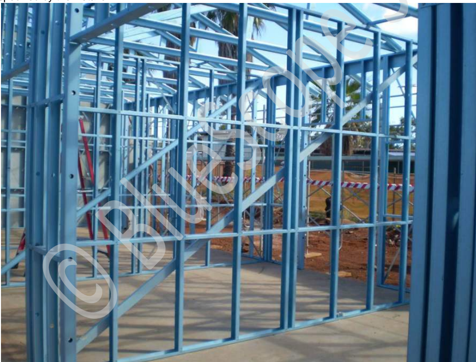
Figure 7.15 Position final wall.
