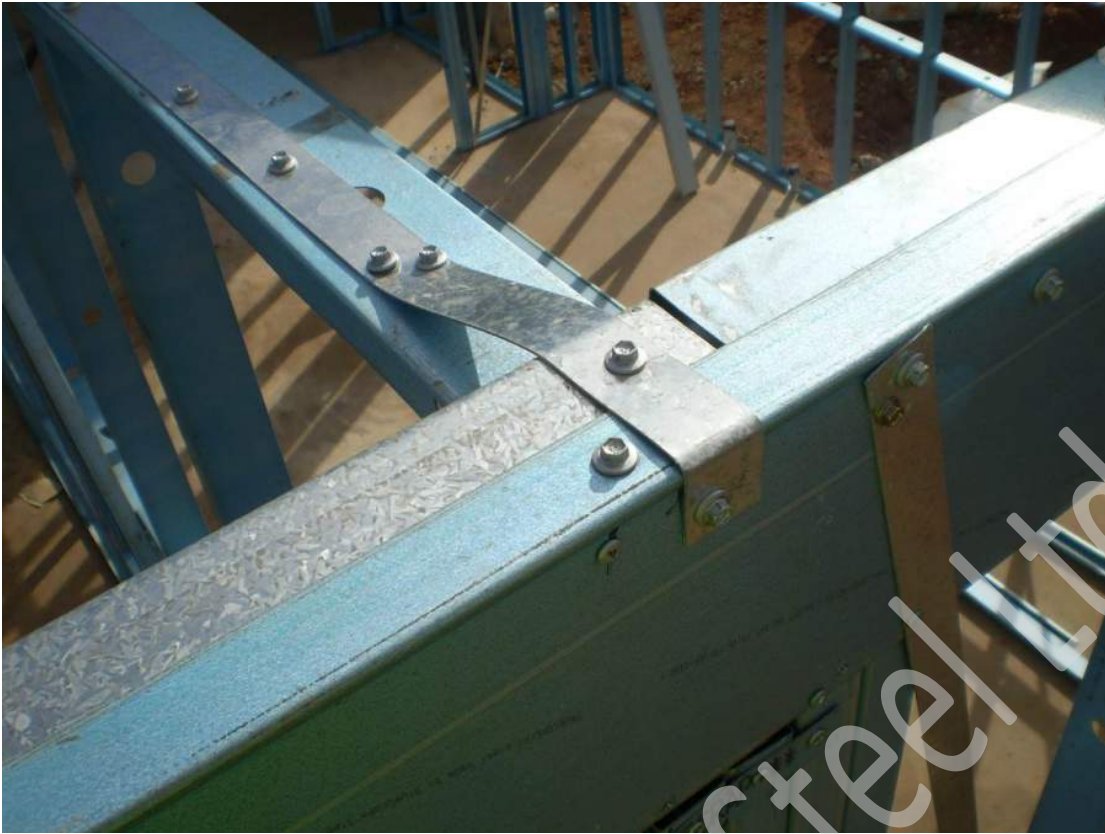
Figure 7.35 Internal to external fixing connections (Option 1)
