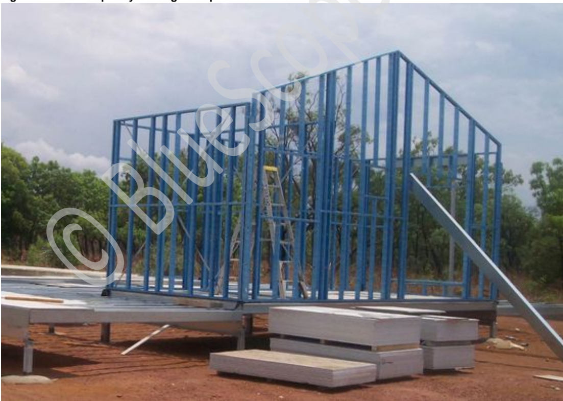
Figure 7.9 Structure with temporary bracing.
