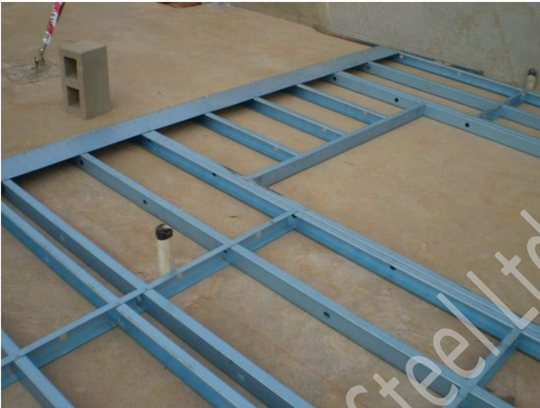
Completed wall frames to be stacked in a flat area ready for installation.
