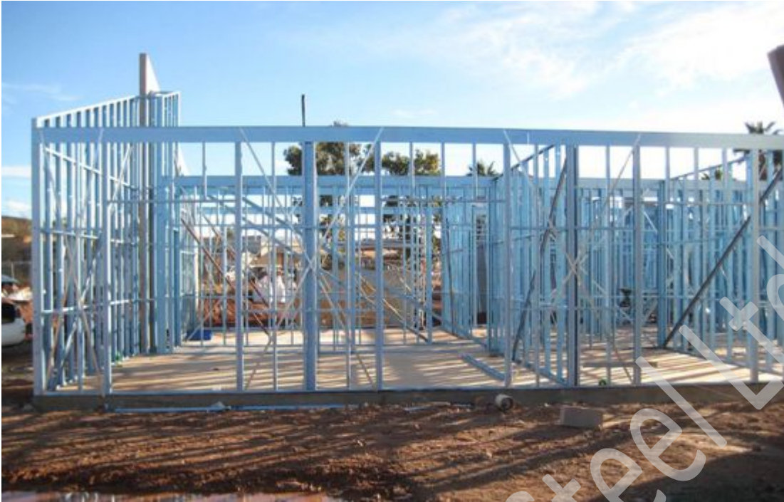
Figure 7.11 Interior walls are fixed into position.
