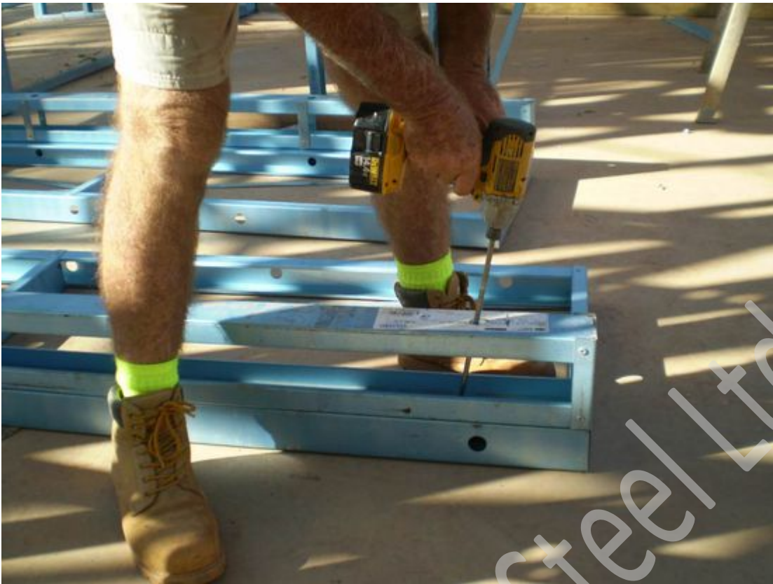
Figure 7.17 Join walls at corner using extension bit.
