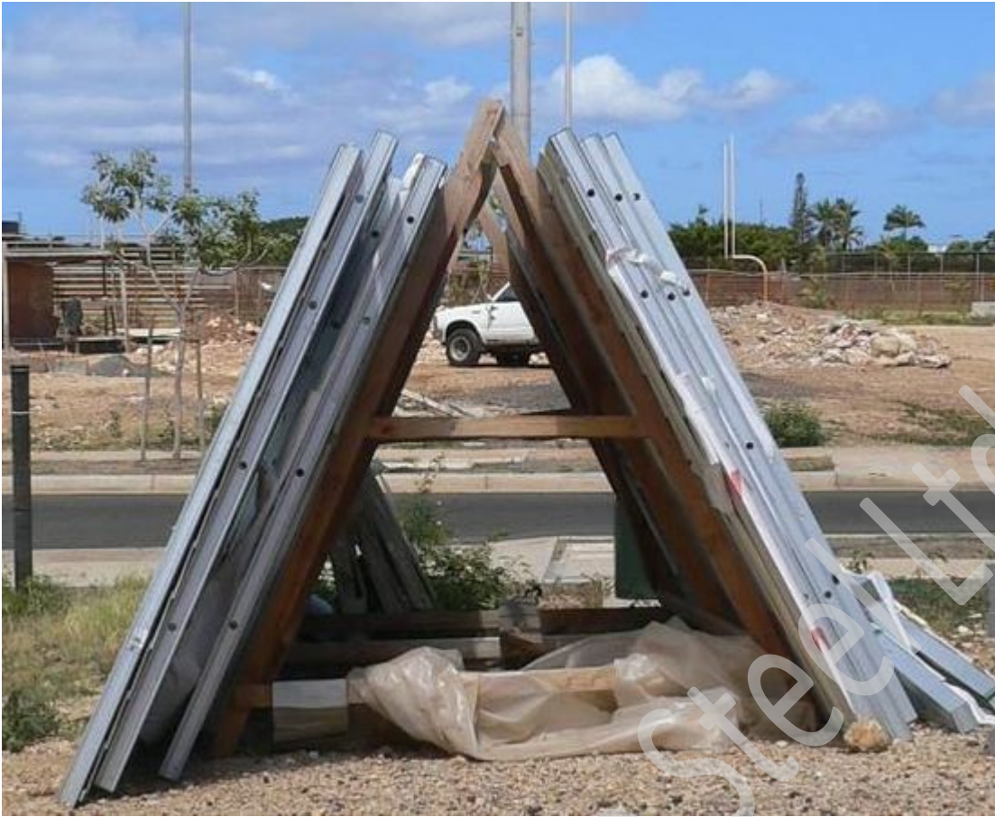
Figure 2.2.1 Frames stacked vertically
