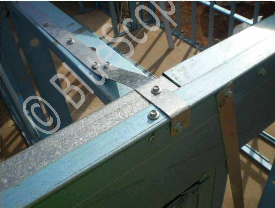
Figure 7.35 Internal to external fixing connections (Option 1)
