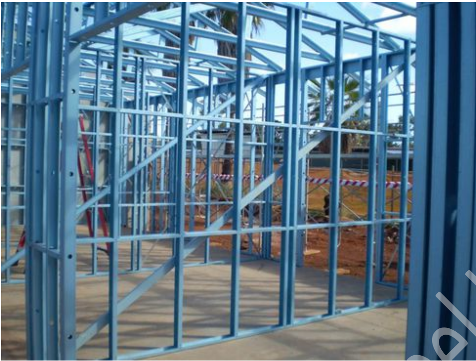
Figure 7.15 Position final wall.
