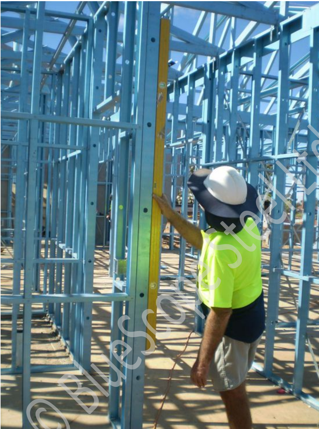
Figure 7.21 Check walls for plumb.
