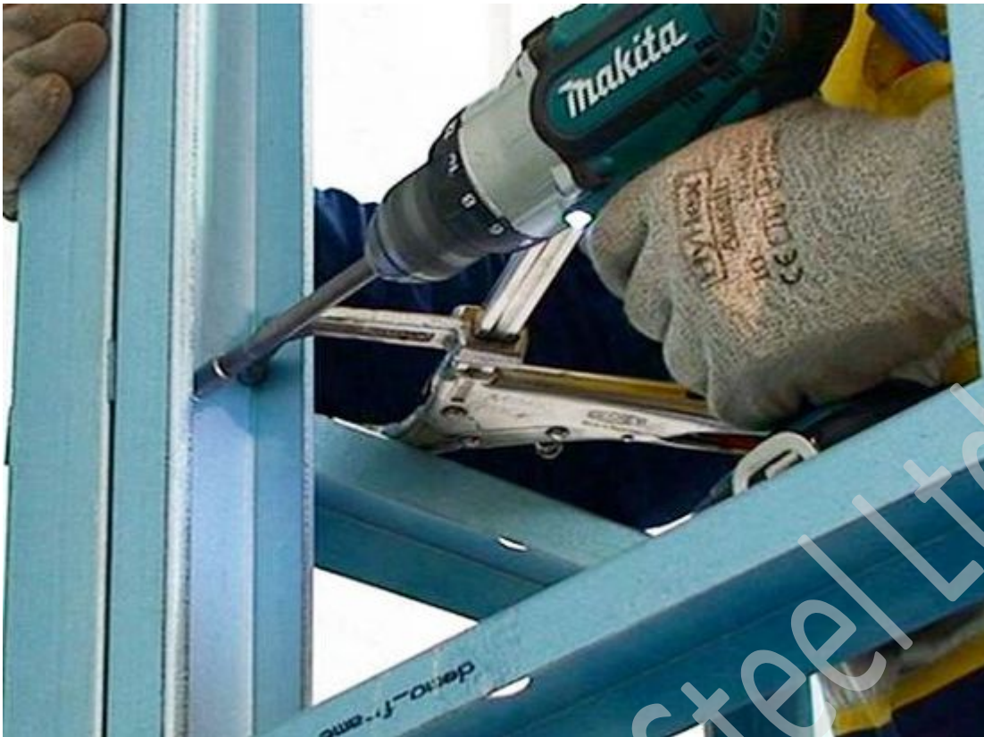
Figure 7.13 End and interior walls are fixed into position.
