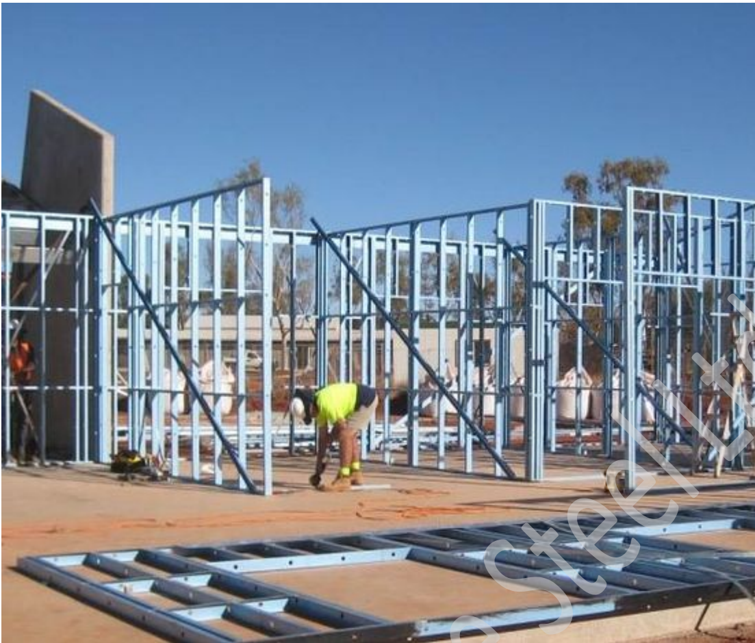
Figure 7.8 Affix temporary bracing as required.
