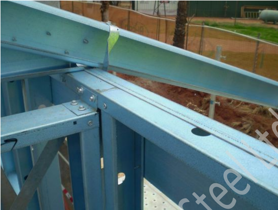
Figure 7.36 Internal to external fixing connections (Option 2)
