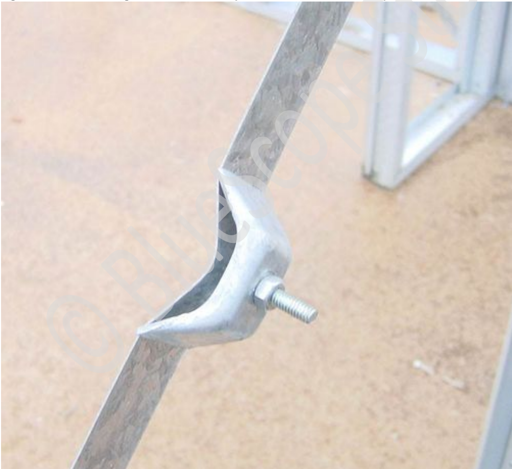
Figure 7.23 use tensioner on strap bracing to bring the wall into square.
