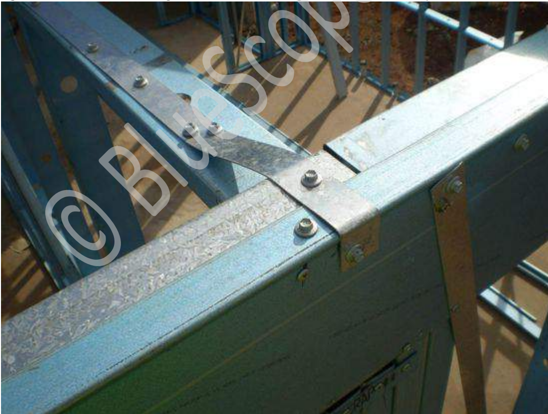
Figure 7.35 Internal to external fixing connections (Option 1)
