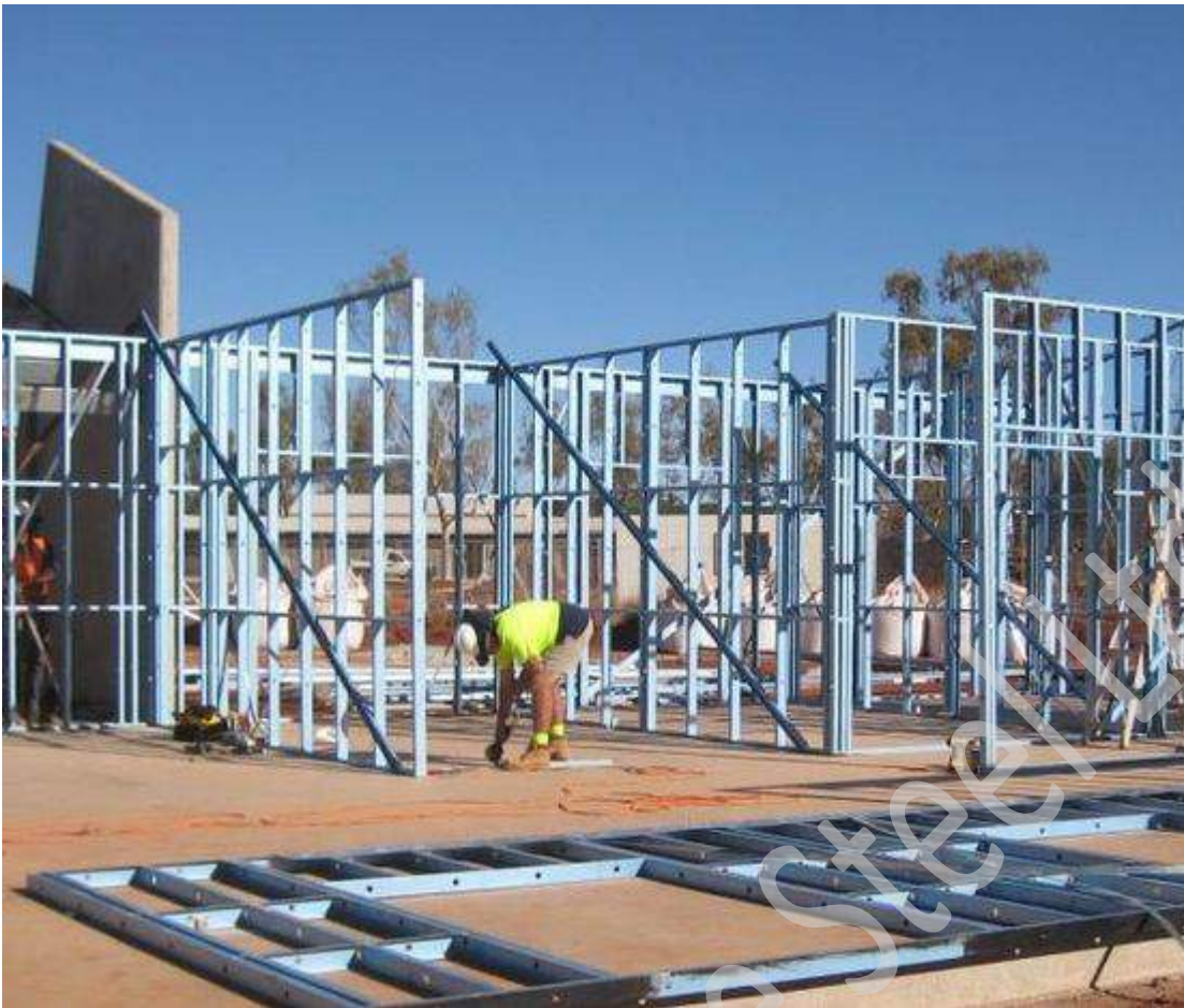
Figure 7.8 Affix temporary bracing as required.
