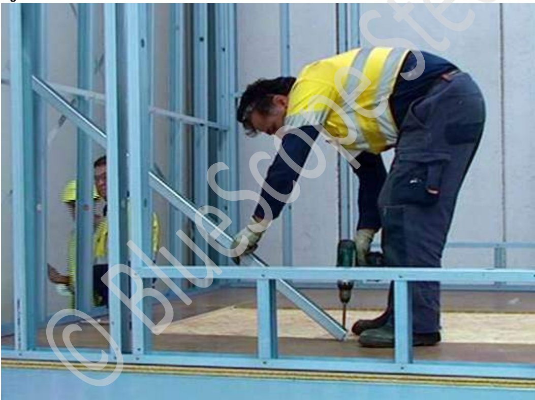
Figure 7.16 Remove last of the temporary bracing.
