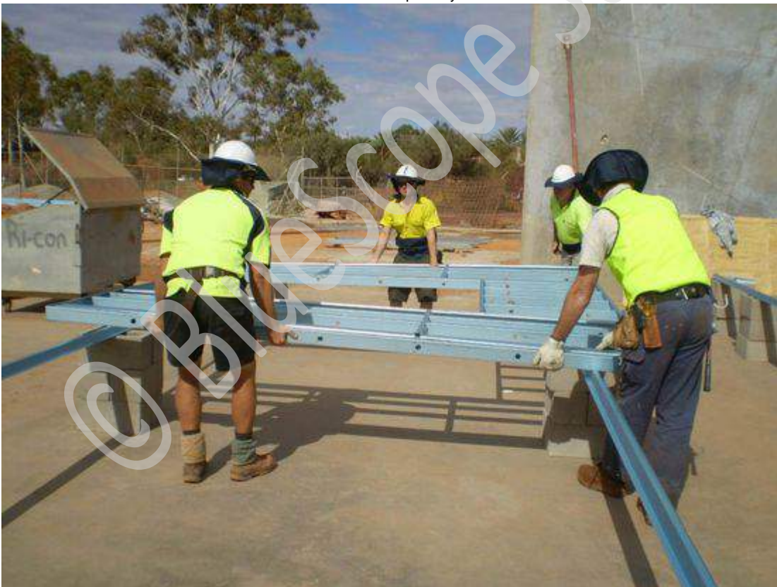
By utilizing two adjoining assembly tables, wall fabrication can be optimized by preparing the next frame while screw fixing & checking "Side B".
