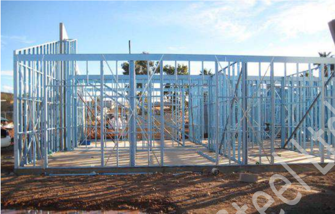
Figure 7.11 Interior walls are fixed into position.
