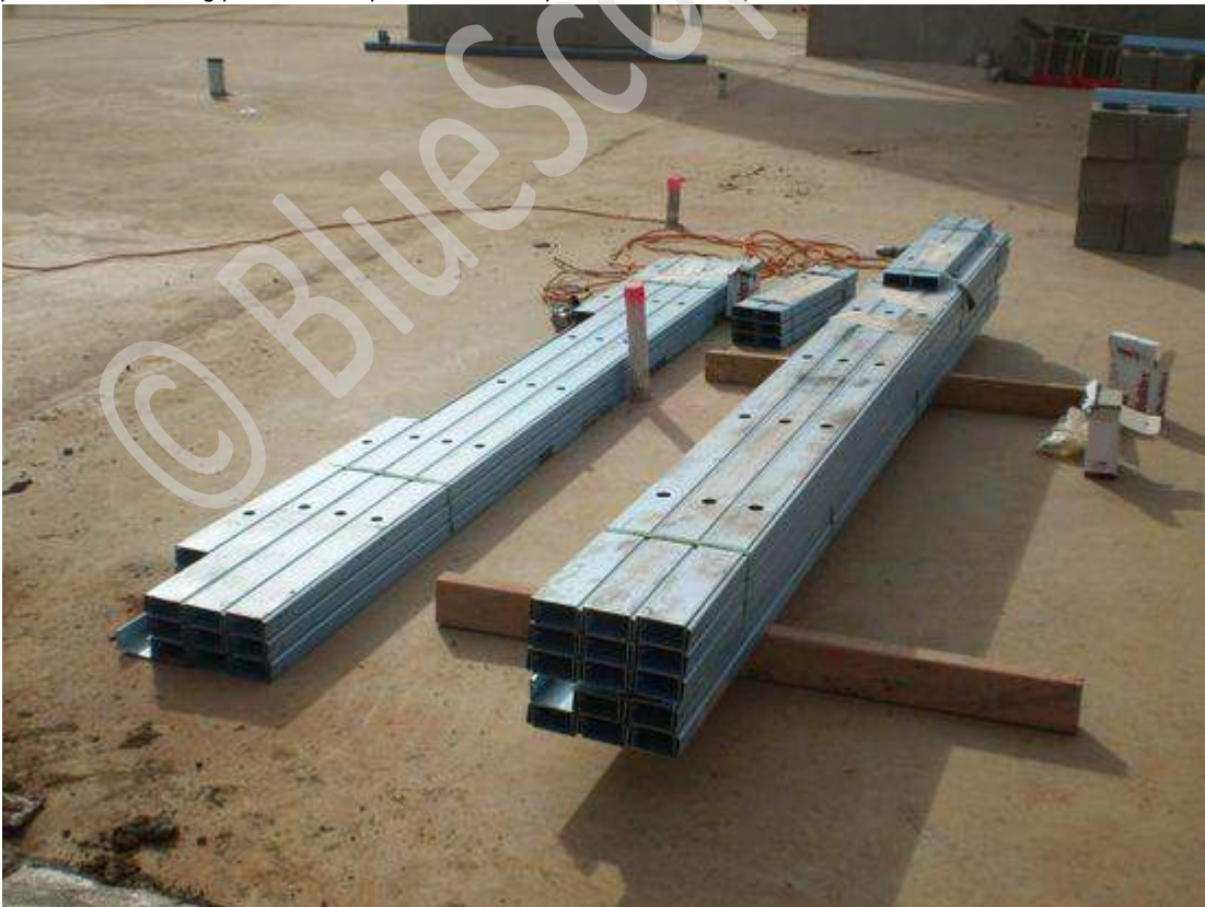
Locate & open matching stud & nogging / plate bundles before separating into individual frame packs.
