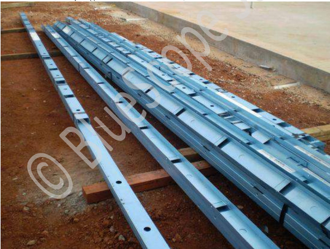
Matching frames in "nogging, top & bottom plate" bundles, labelled with bundle numbers
