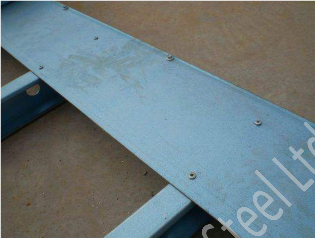
Overlay & screw fix lintel flashing to top of frame as per assembly sheet & fixing details given in the Design Manual.
