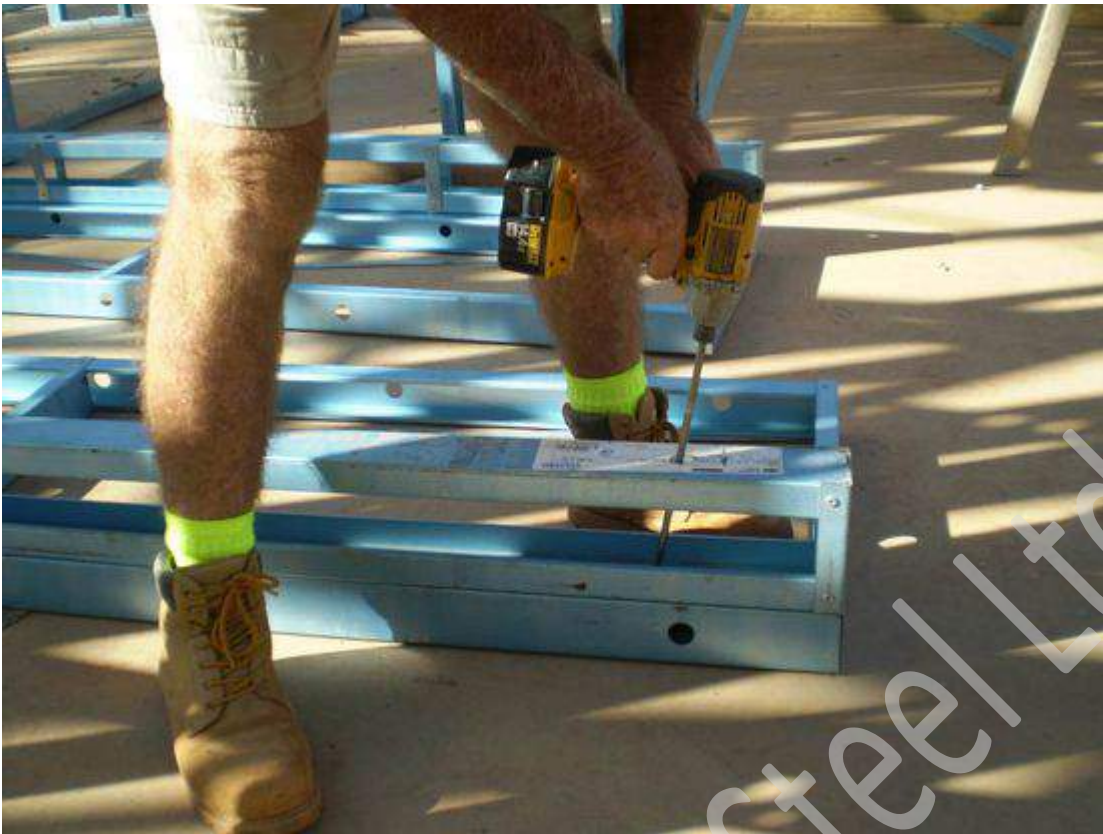
Figure 7.17 Join walls at corner using extension bit.
