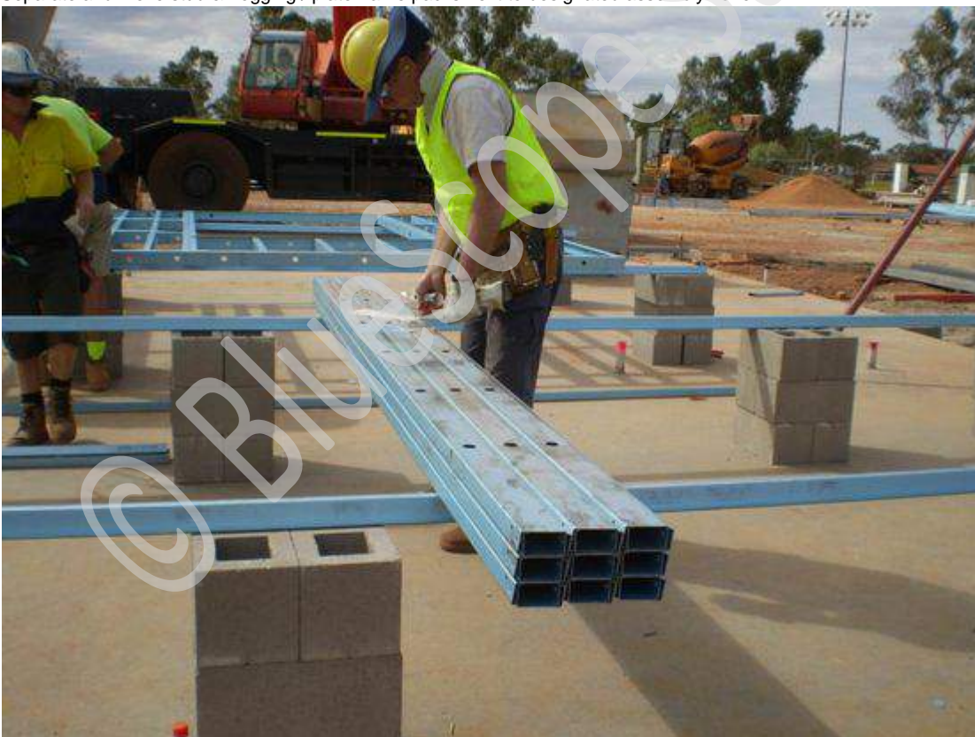
Lift & separate stud pack onto assembly table (this example has utilised Topspan ® 40 sections on concrete block stacks as an assembly table).
