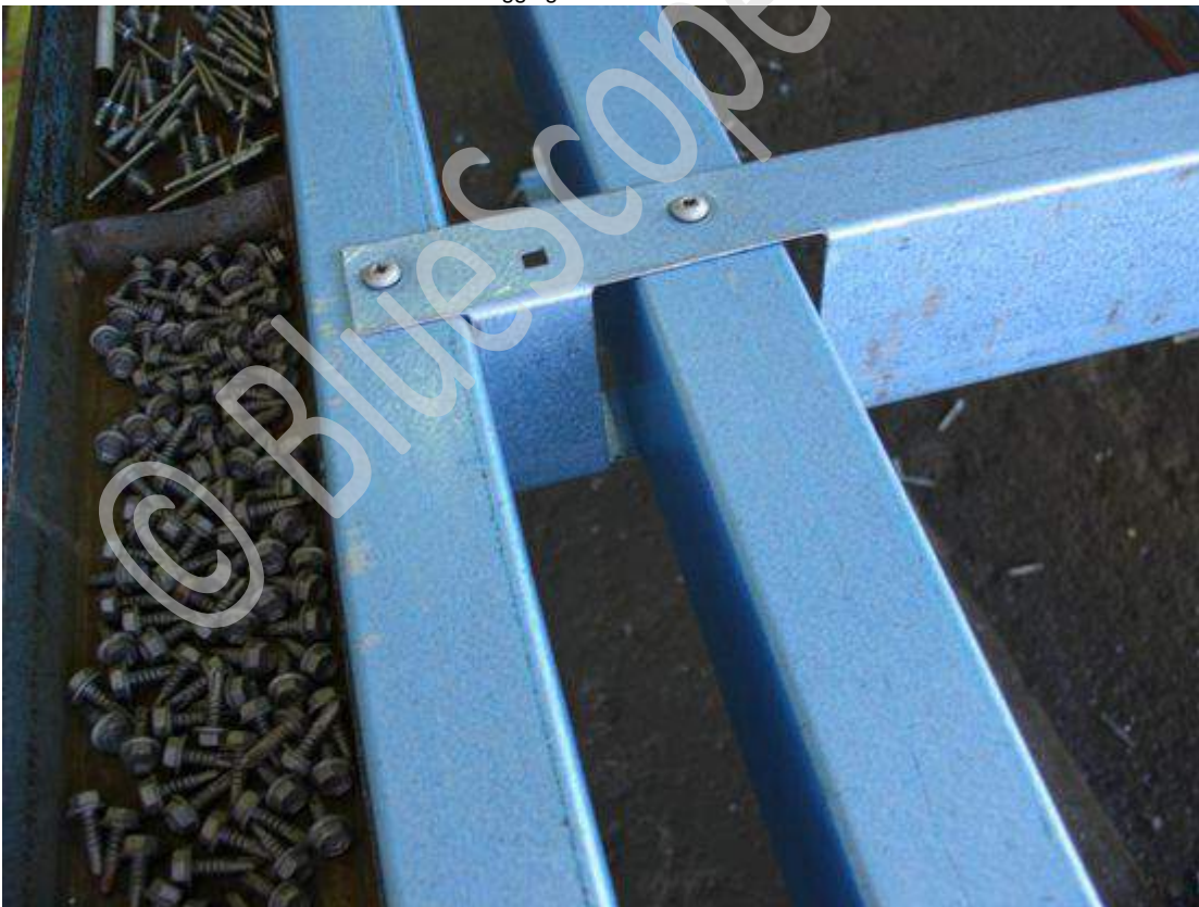
Nogging installation.
