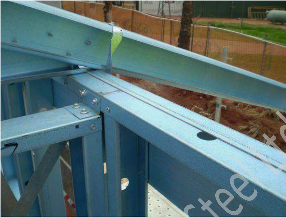
Figure 7.36 Internal to external fixing connections (Option 2)
