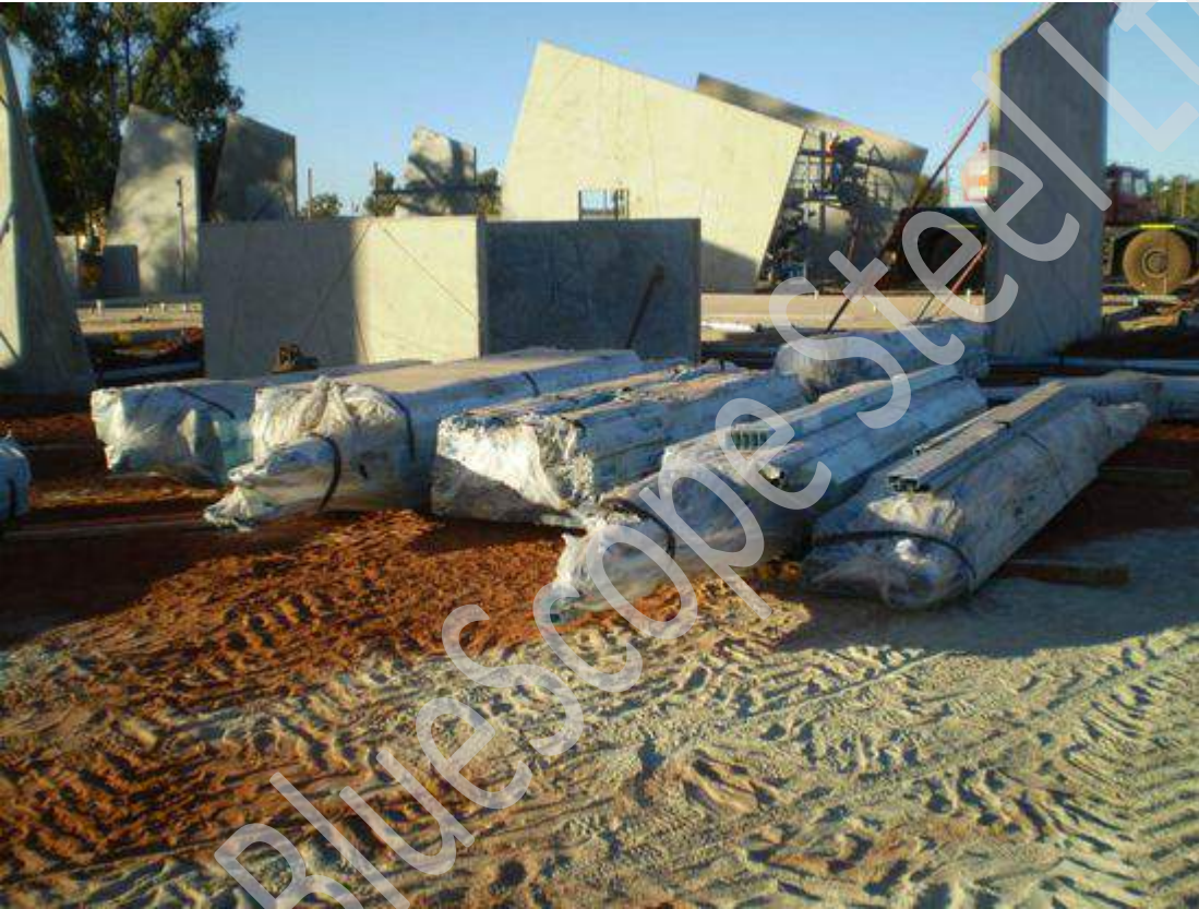
Wall & truss framing will be plastic wrapped & labelled in bundles as registered on packing list
