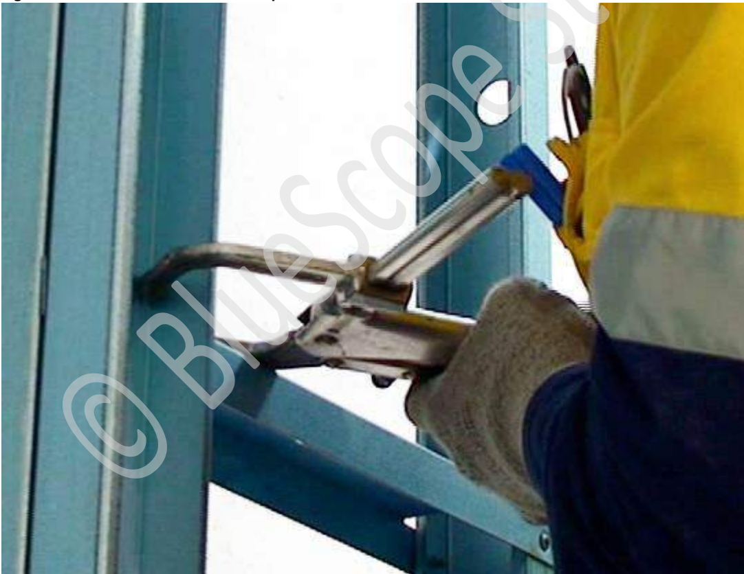
Figure 7.12 Use clamp to hold temporarily in position.
