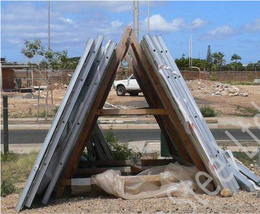
Figure 2.2.1 Frames stacked vertically
