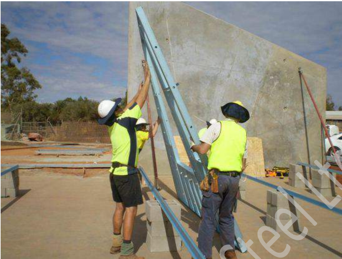
Ensure sufficient labour available on both sides of frame to flip safely.
