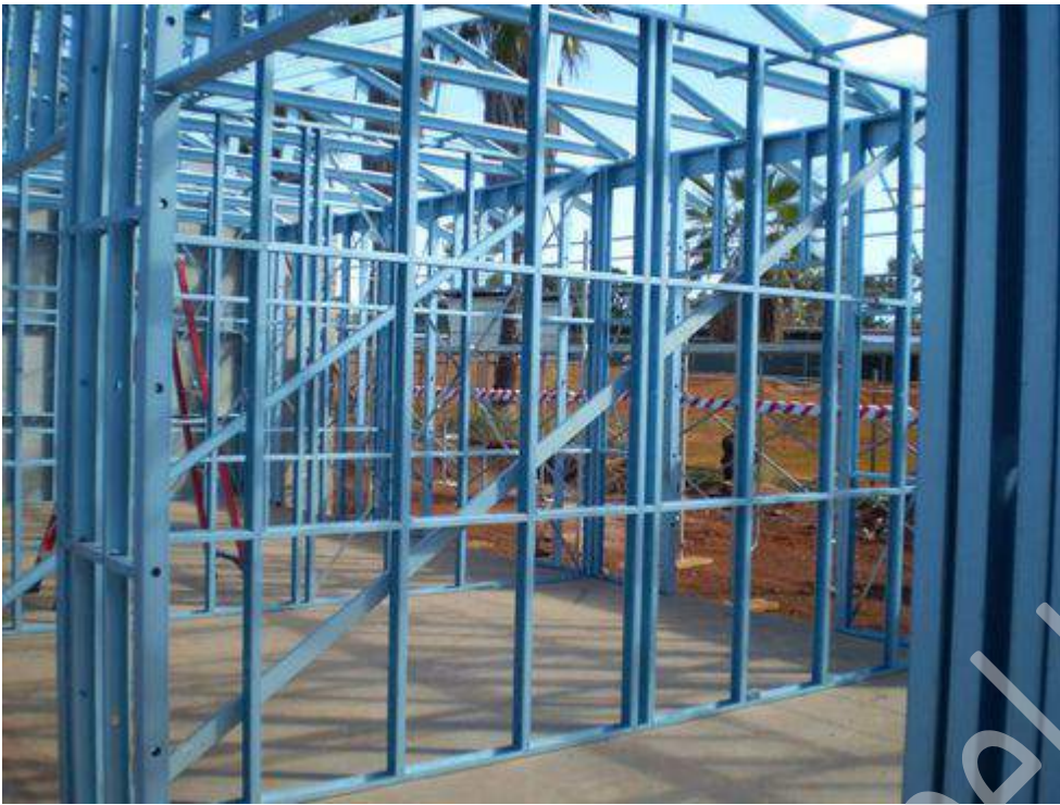
Figure 7.15 Position final wall.
