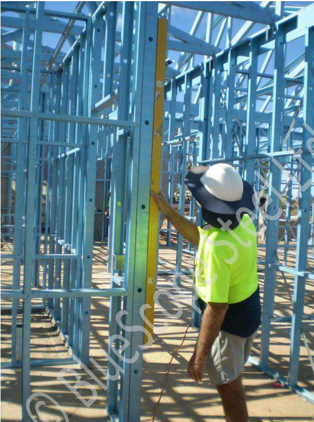
Figure 7.21 Check walls for plumb.
