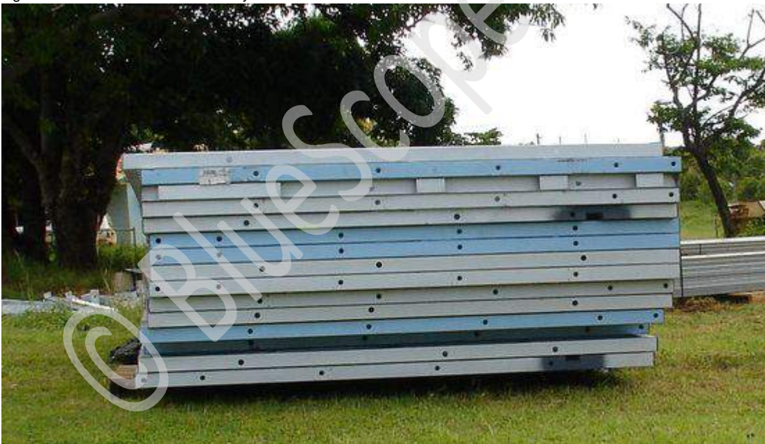
Figure 2.2.2 Frames stacked horizontally
