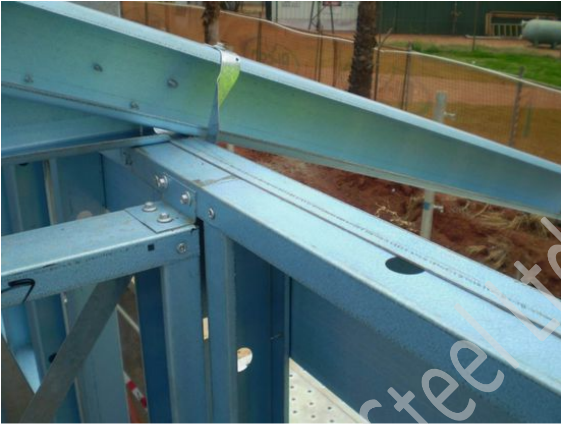
Figure 7.36 Internal to external fixing connections (Option 2)
