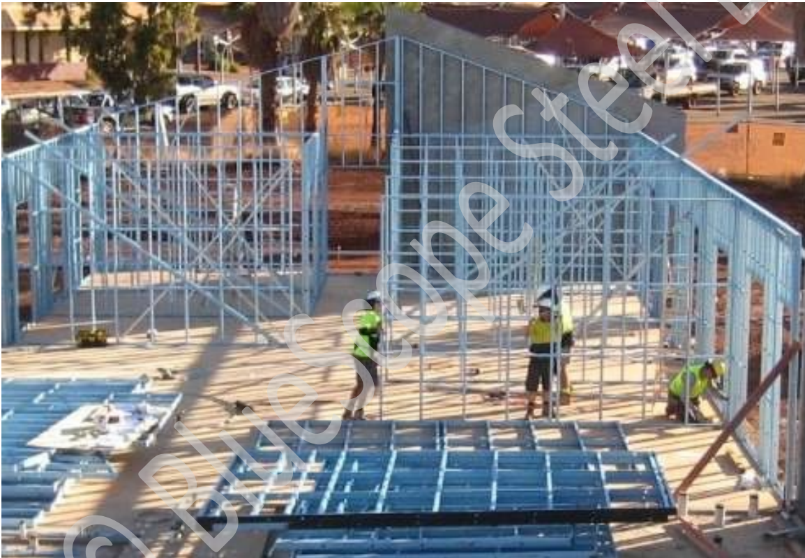
Stack wall frames in bundles close to the final installation position.
