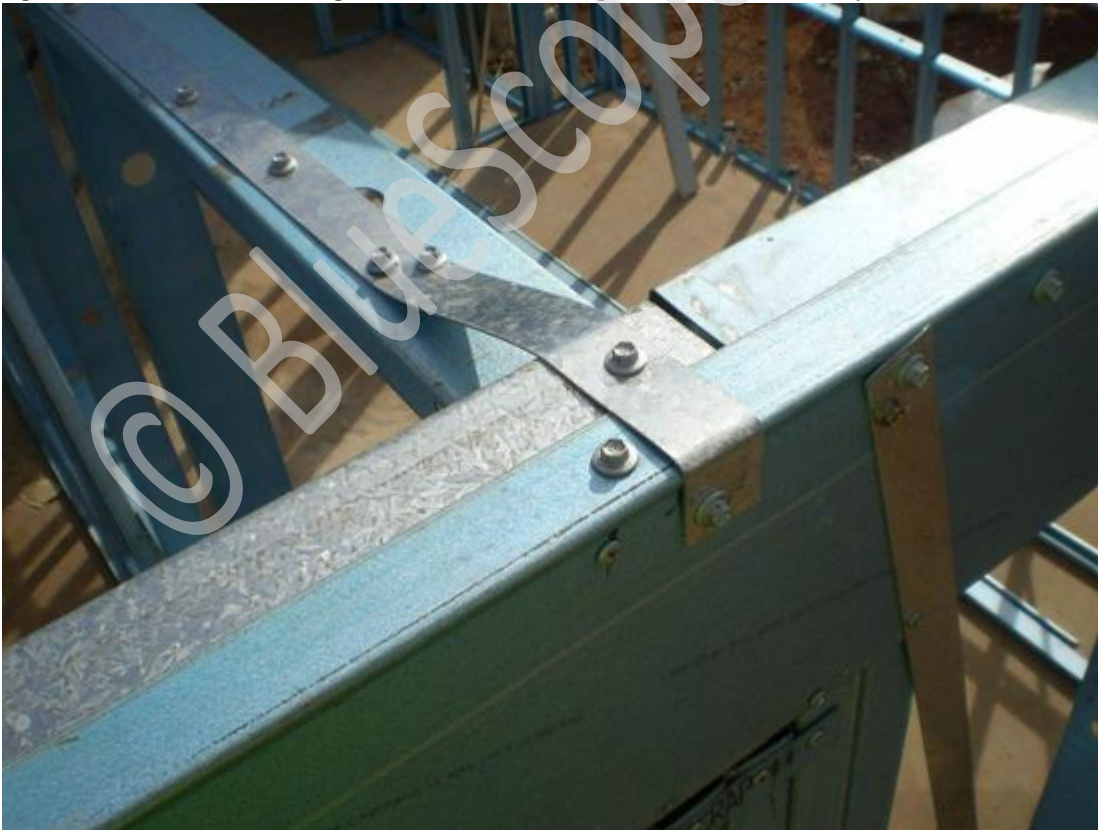
Figure 7.35 Internal to external fixing connections (Option 1)
