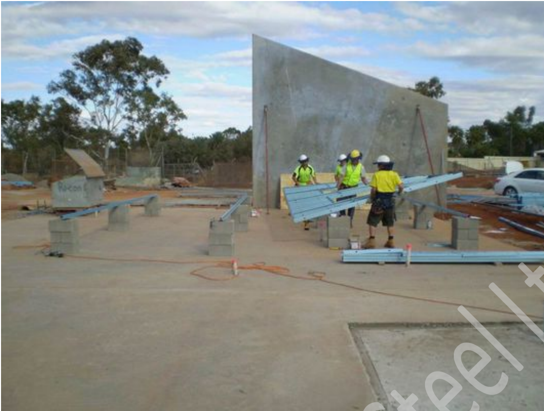
Cross check "Side A" frame layout & connections as per assembly sheet. Utilizing sufficient labour, lift & flip frame for "Side B" screw fixings.
