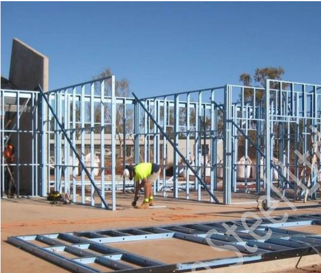
Figure 7.8 Affix temporary bracing as required.
