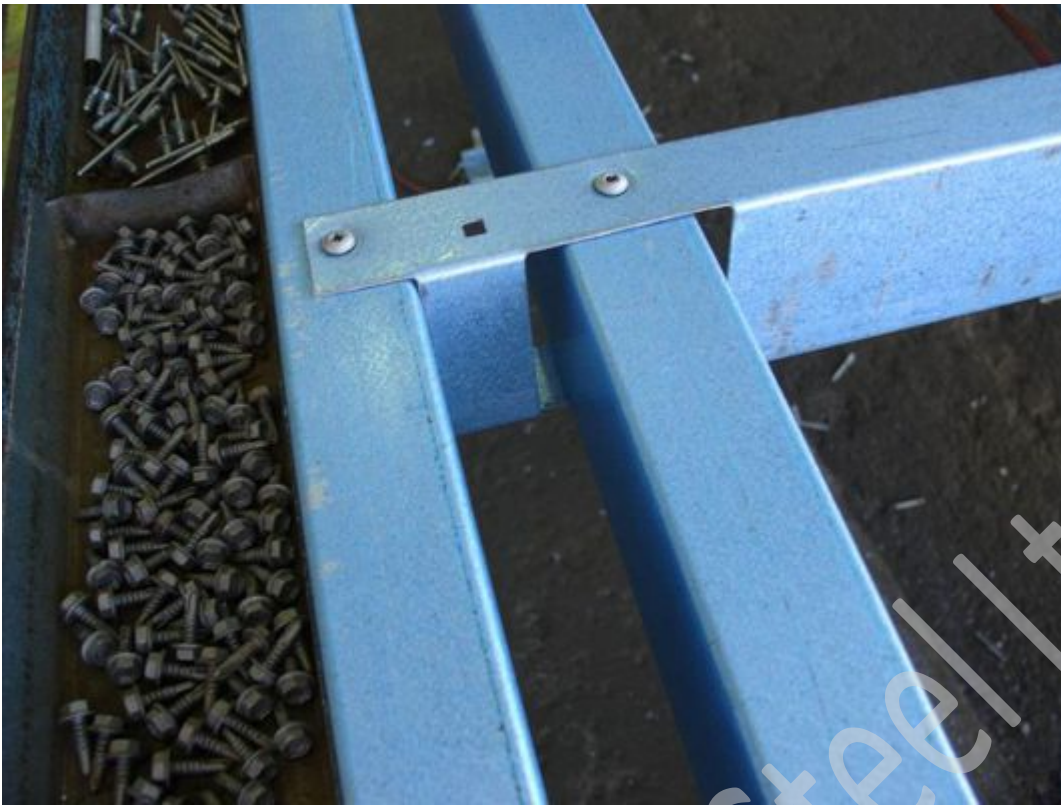
Nogging installation.
