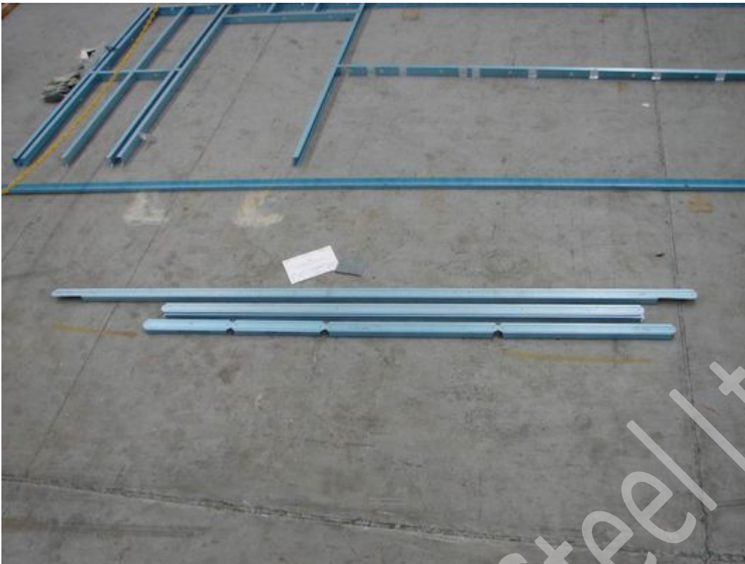
Separate and move stud & nogging / plate frame packs next to designated assembly zone.
