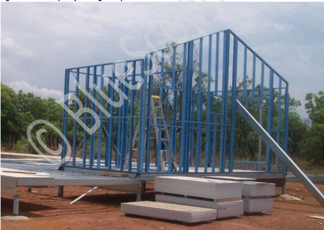
Figure 7.9 Structure with temporary bracing.
