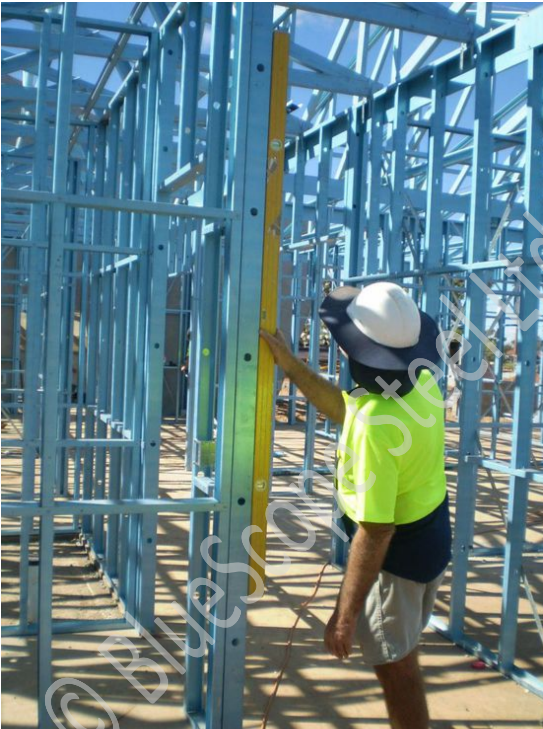
Figure 7.21 Check walls for plumb.
