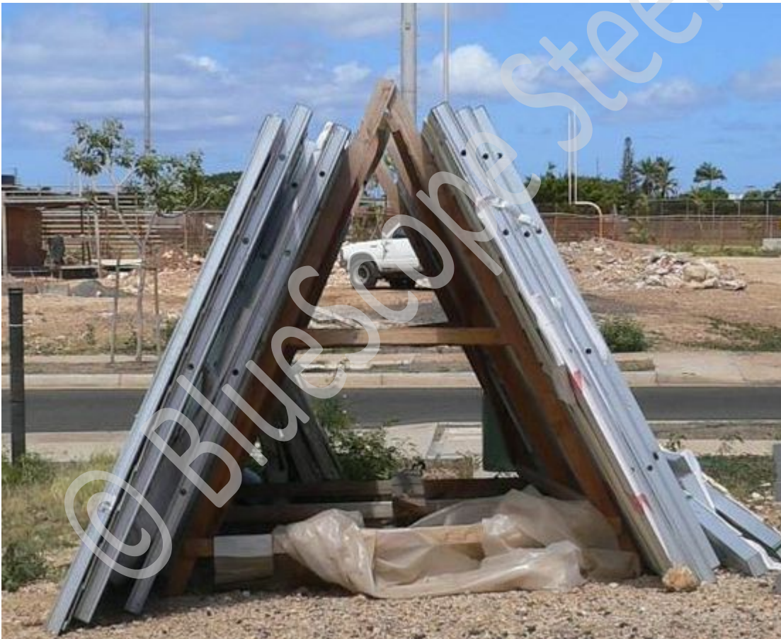
Figure 2.2.1 Frames stacked vertically
