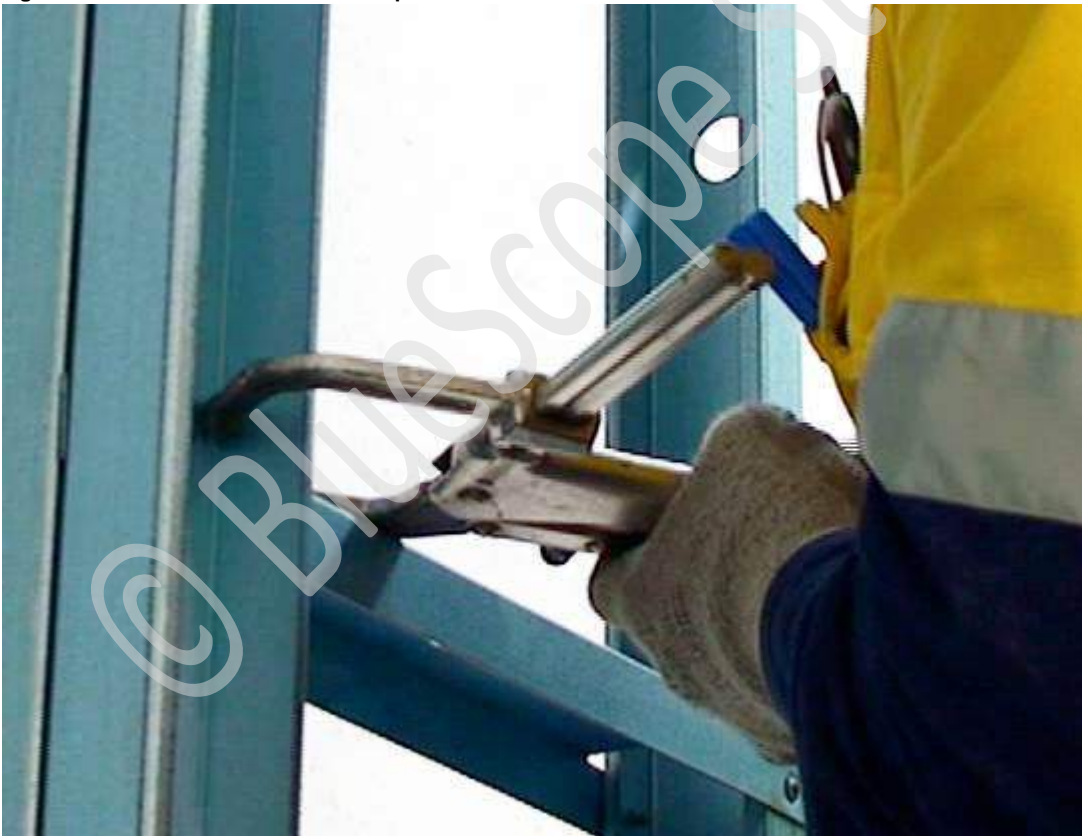
Figure 7.12 Use clamp to hold temporarily in position.
