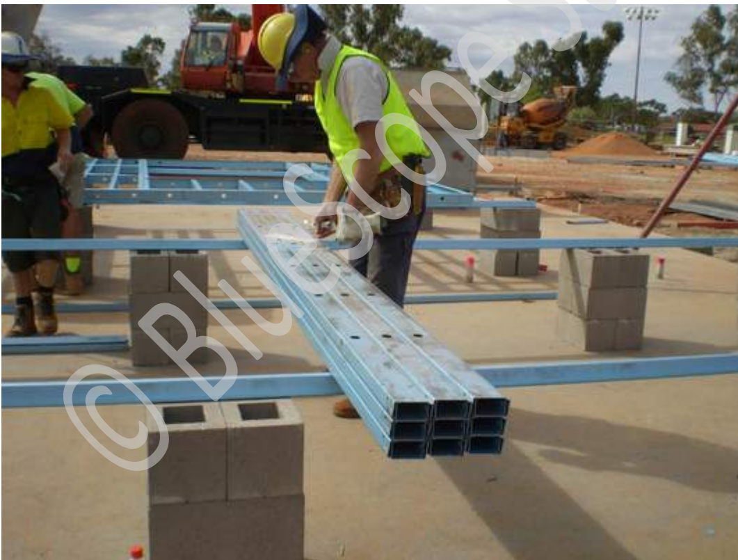
Lift and separate stud pack onto assembly table (this example has utilised Topspan ® 40 sections on concrete block stacks as an assembly table).
