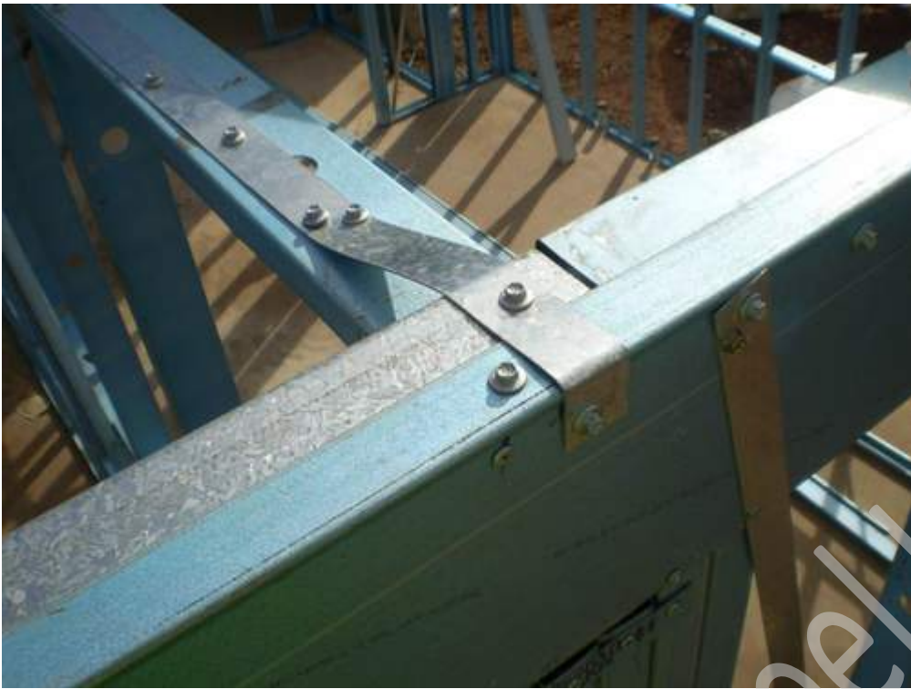
Internal to external fixing connections (Option 2)
