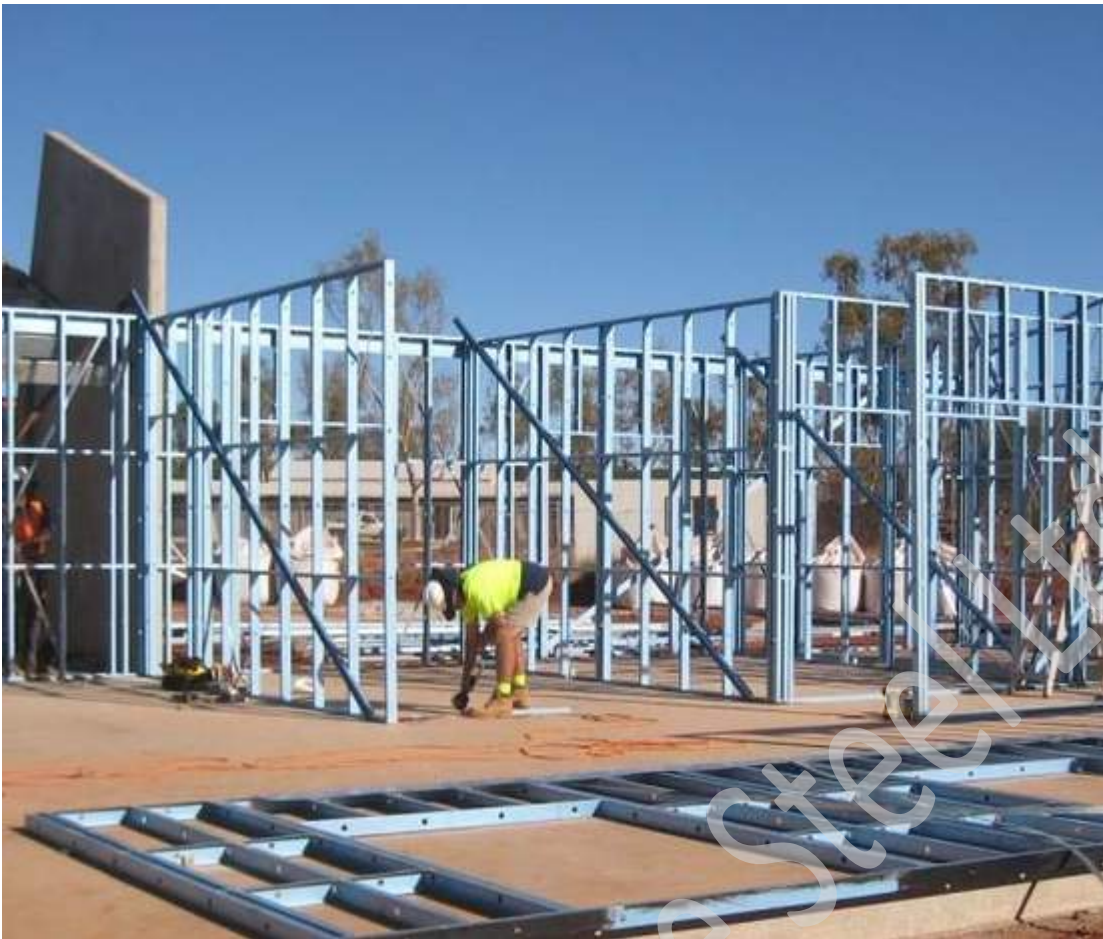
Figure 7.8 Affix temporary bracing as required.
