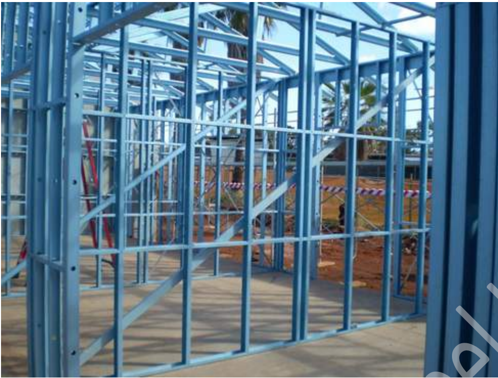
Figure 7.15 Position final wall.
