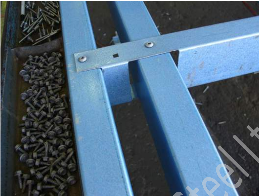
Nogging installation.
