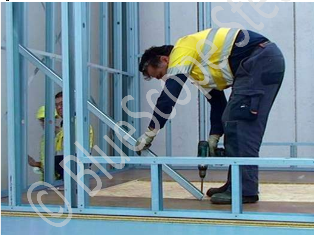
Figure 7.16 Remove last of the temporary bracing.
