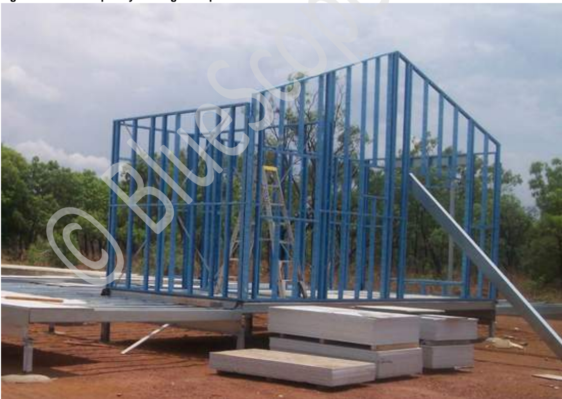
Figure 7.9 Structure with temporary bracing.
