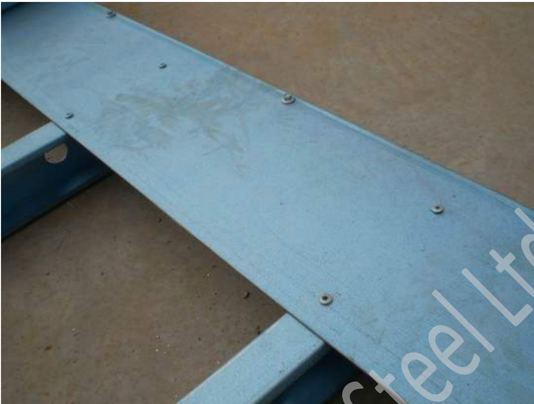
Overlay and screw fix lintel flashing to top of frame as per assembly sheet and fixing details given in the Design Manual.
