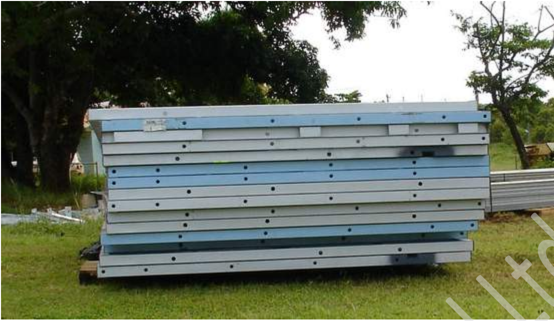
Figure 2.2.2 Frames stacked horizontally
