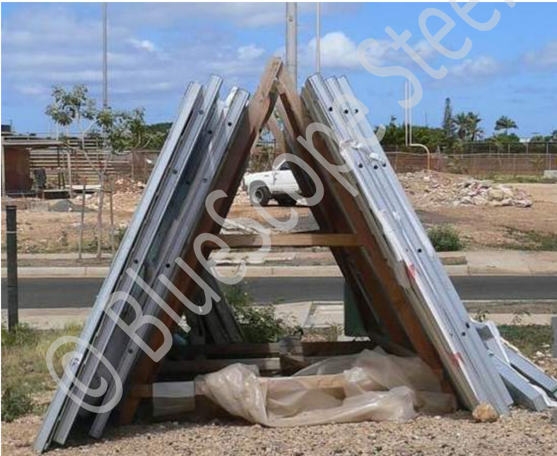
Figure 2.2.1 Frames stacked vertically
