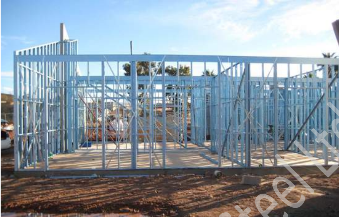
Figure 7.11 Interior walls are fixed into position.
