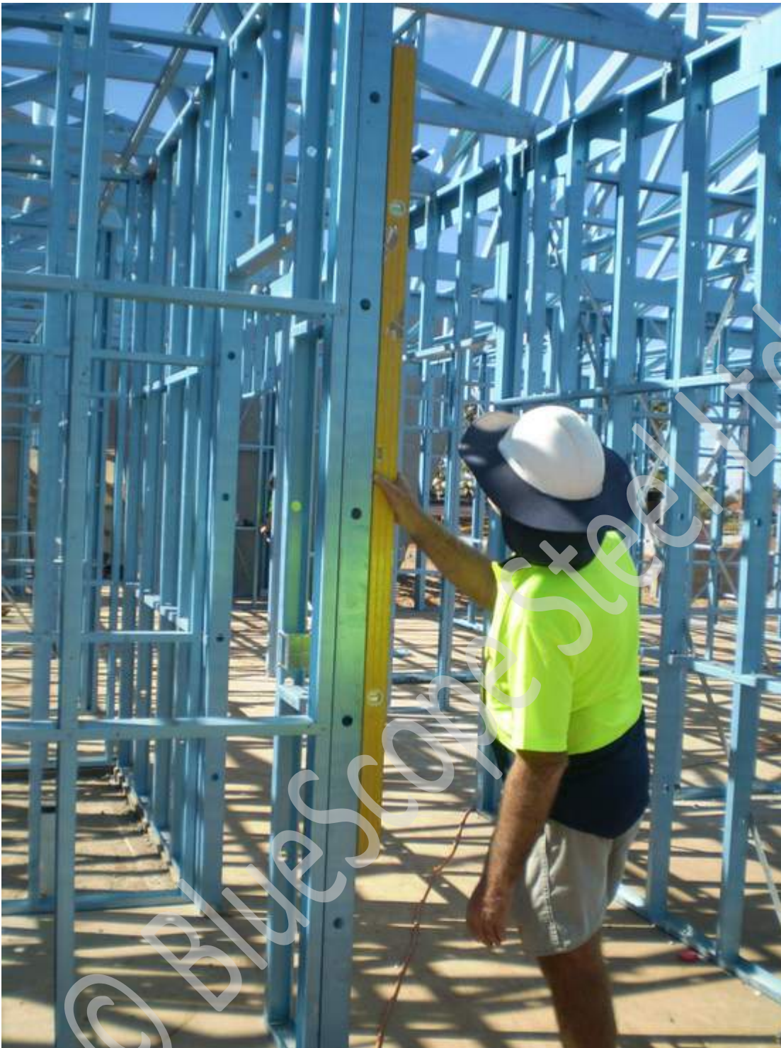
Figure 7.21 Check walls for plumb.
