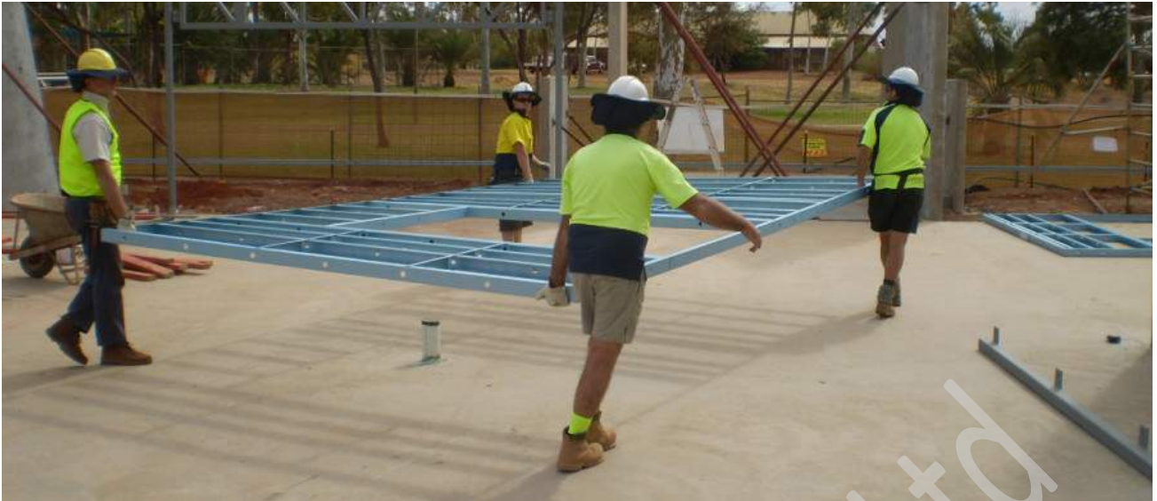
Relocate completed frames to a designated stacking area.
