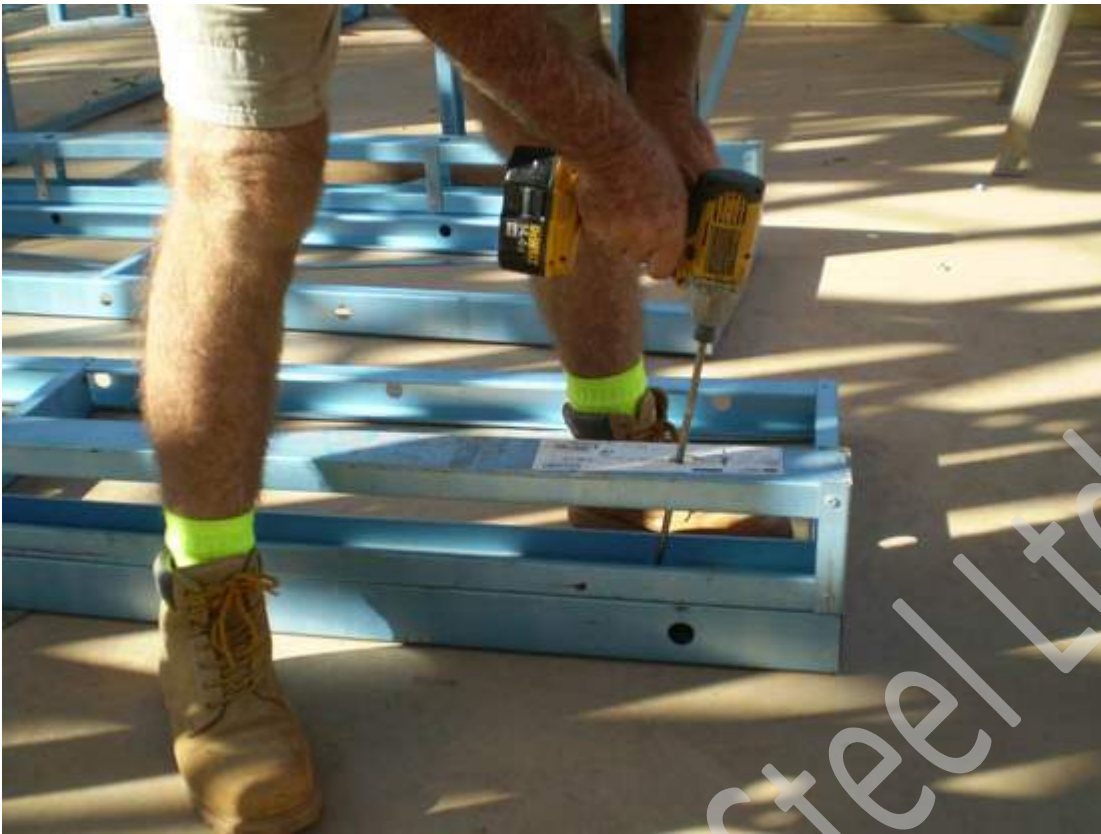
Figure 7.17 Join walls at corner using extension bit.
