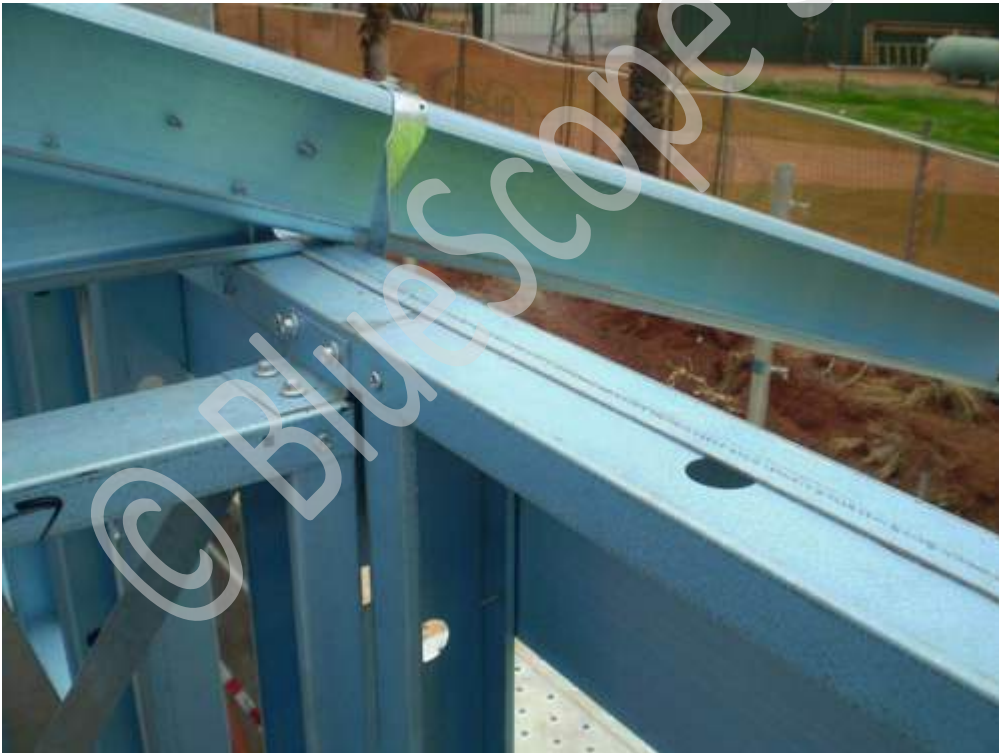
Internal to external fixing connections (Option 2)
