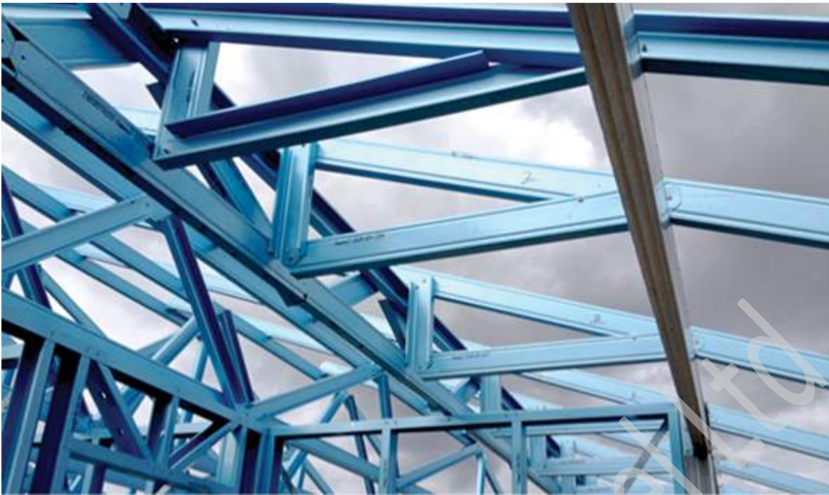
Figure 7.24a Installation of a Type 1A hip truss
