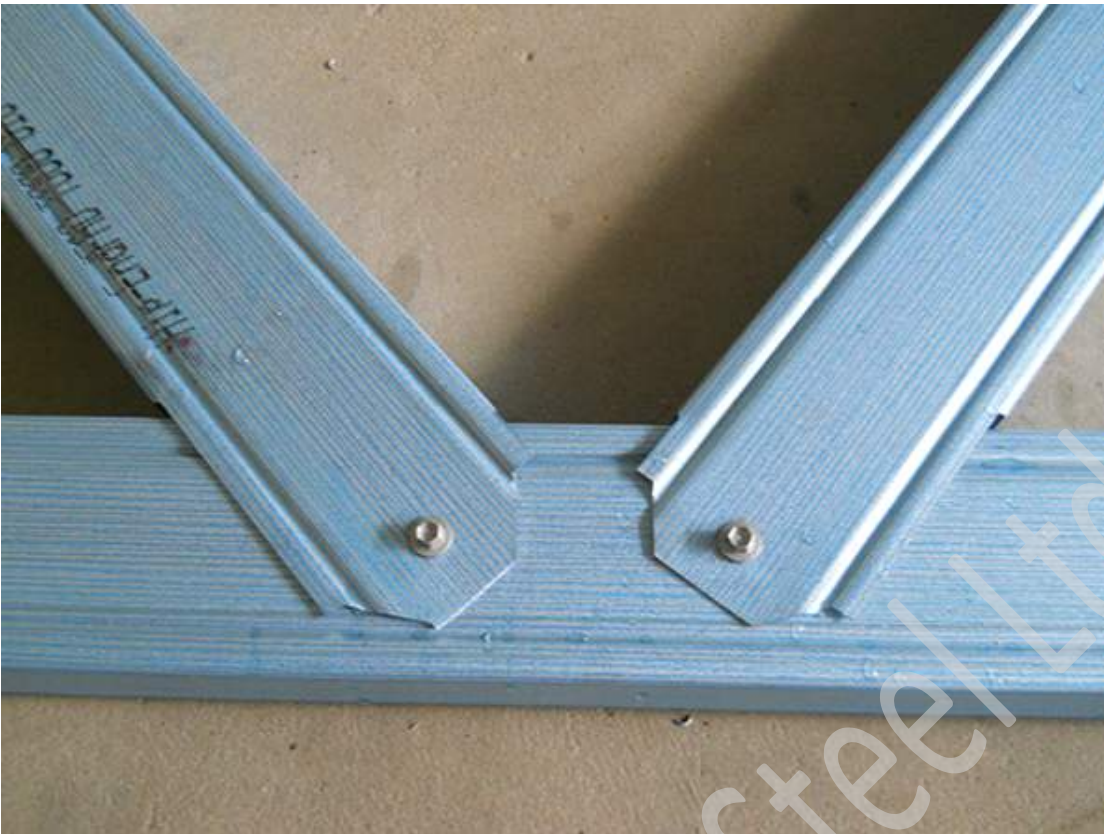
Finished knee web connection (unreinforced)
