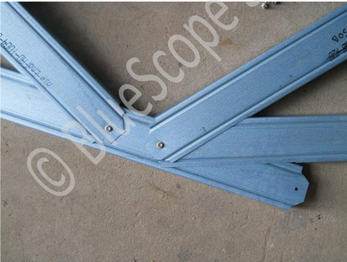
Finished connection (reinforced)
