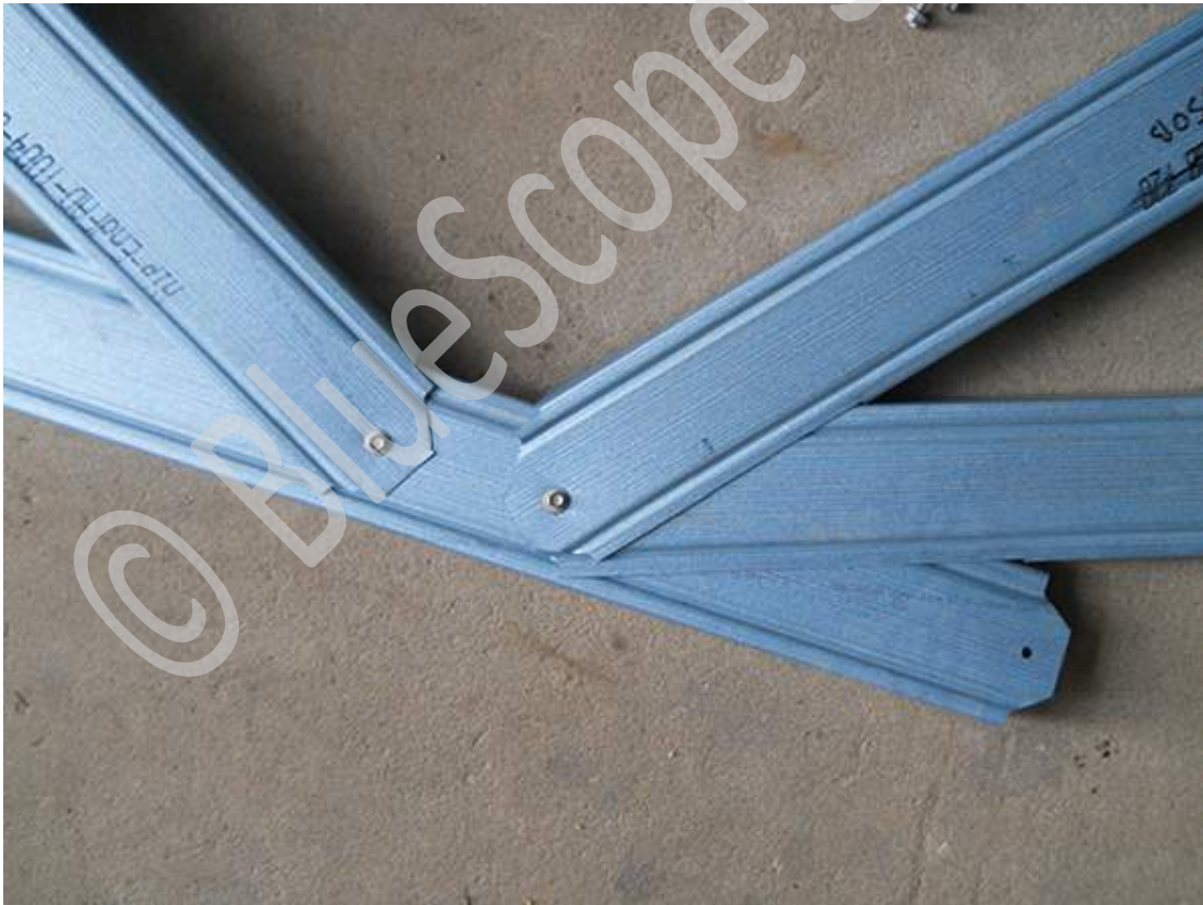
Finished connection (reinforced)
