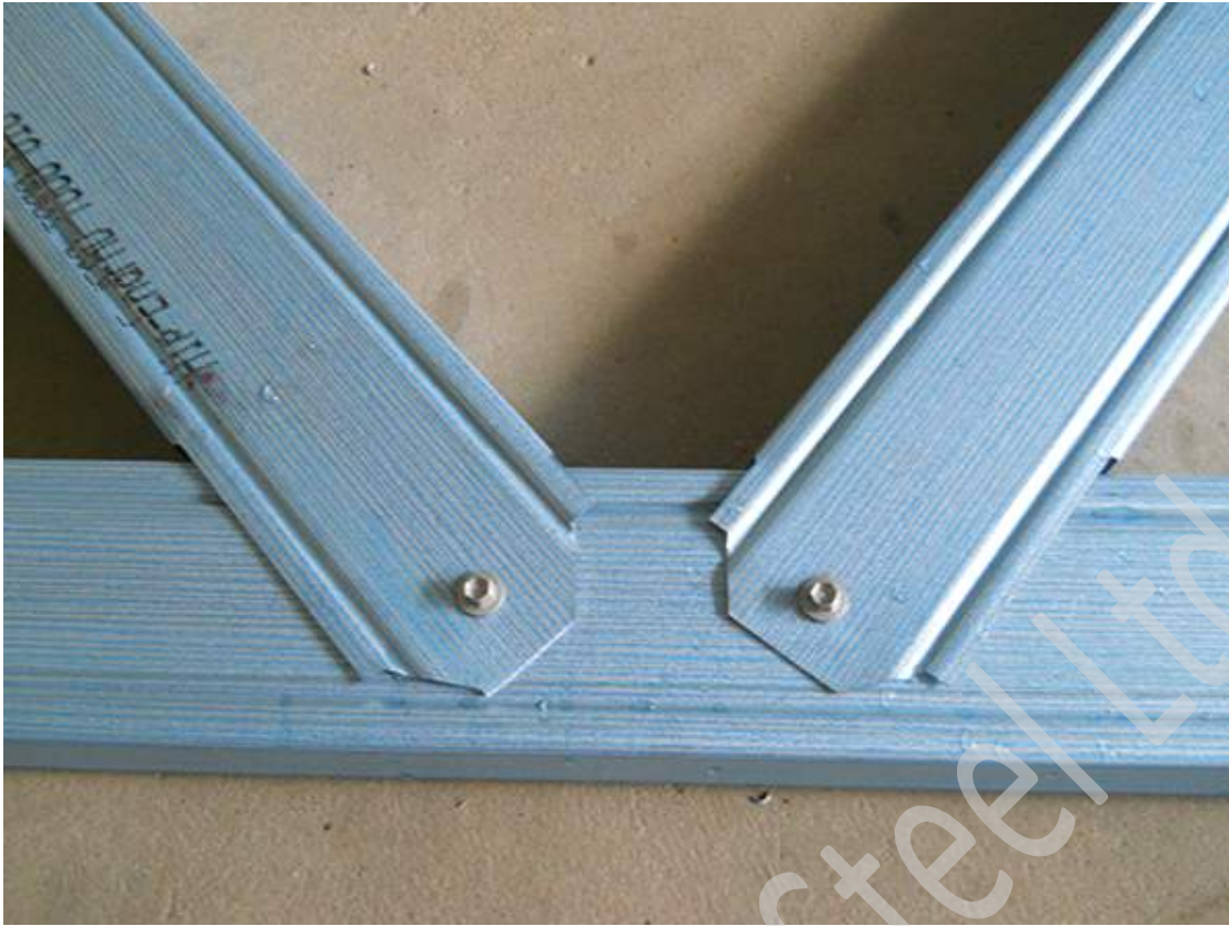
Finished knee web connection (unreinforced)
