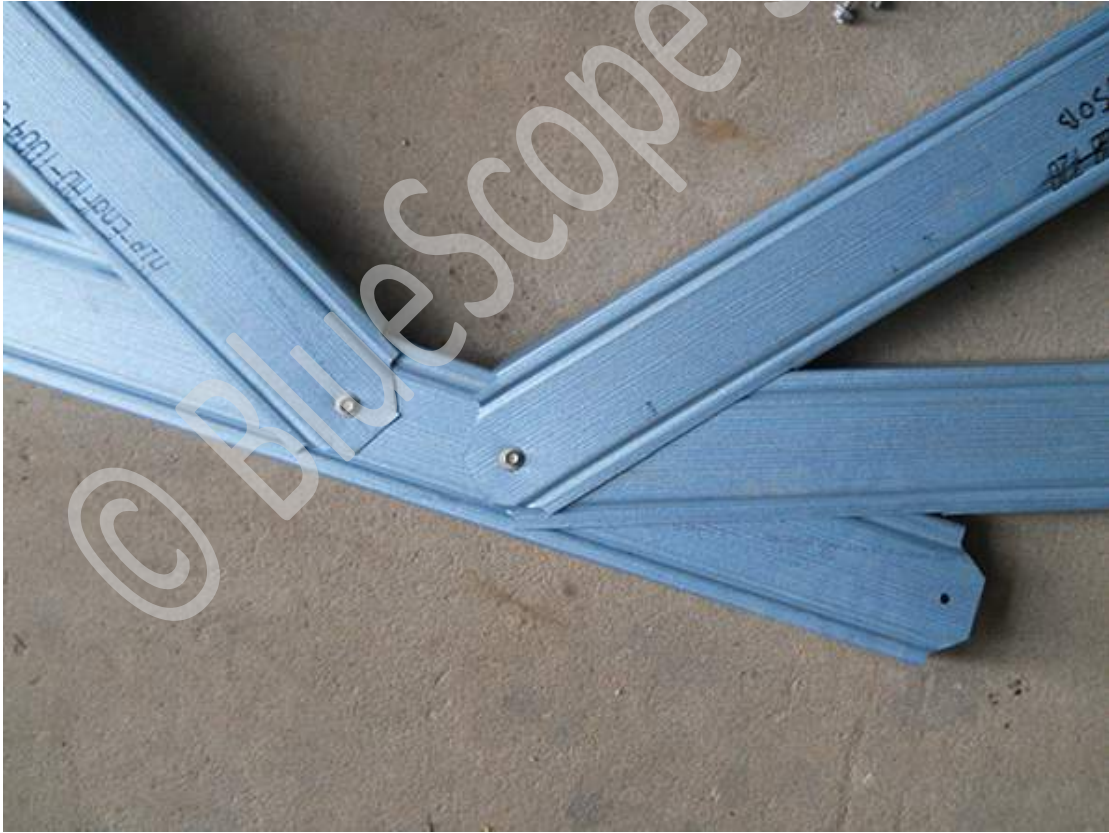
Finished connection (reinforced)
