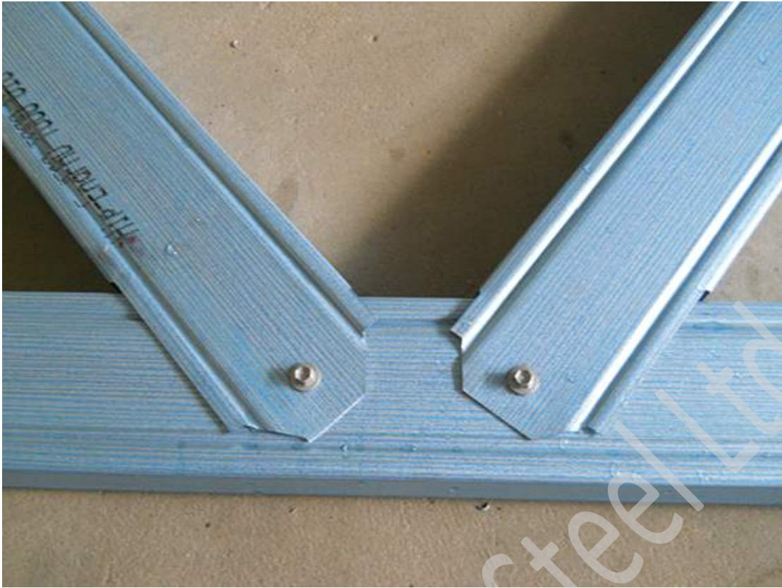
Finished knee web connection (unreinforced)
