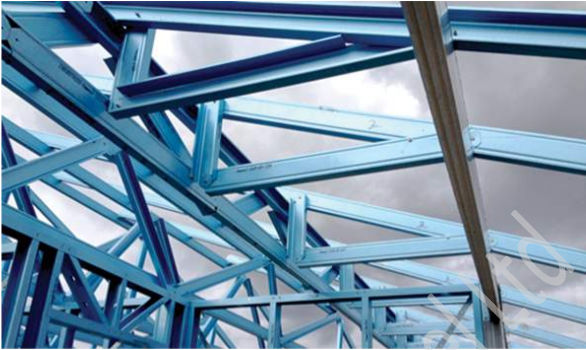
Figure 7.24a Installation of a Type 1A hip truss
