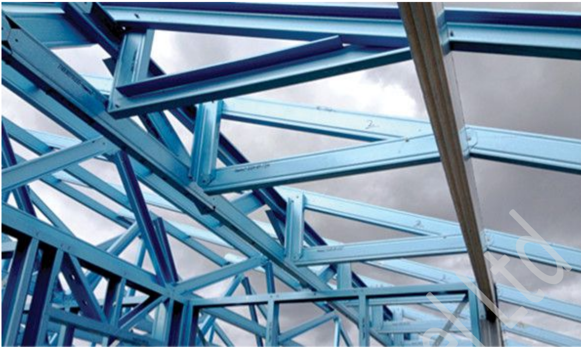
Figure 7.24a Installation of a Type 1A hip truss
