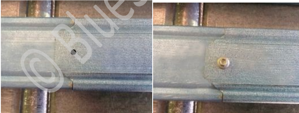
Figure 6.3 Bottom Chord connection at splice
