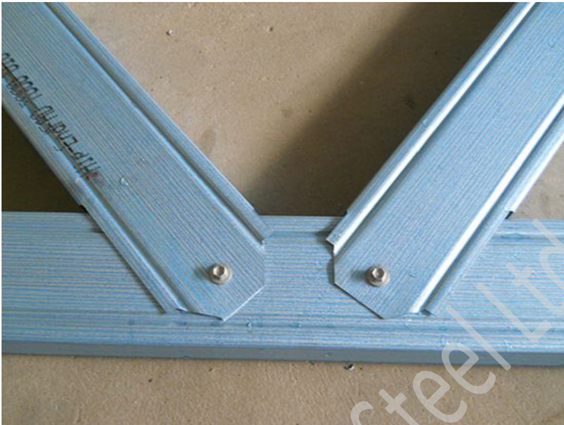
Finished knee web connection (unreinforced)
