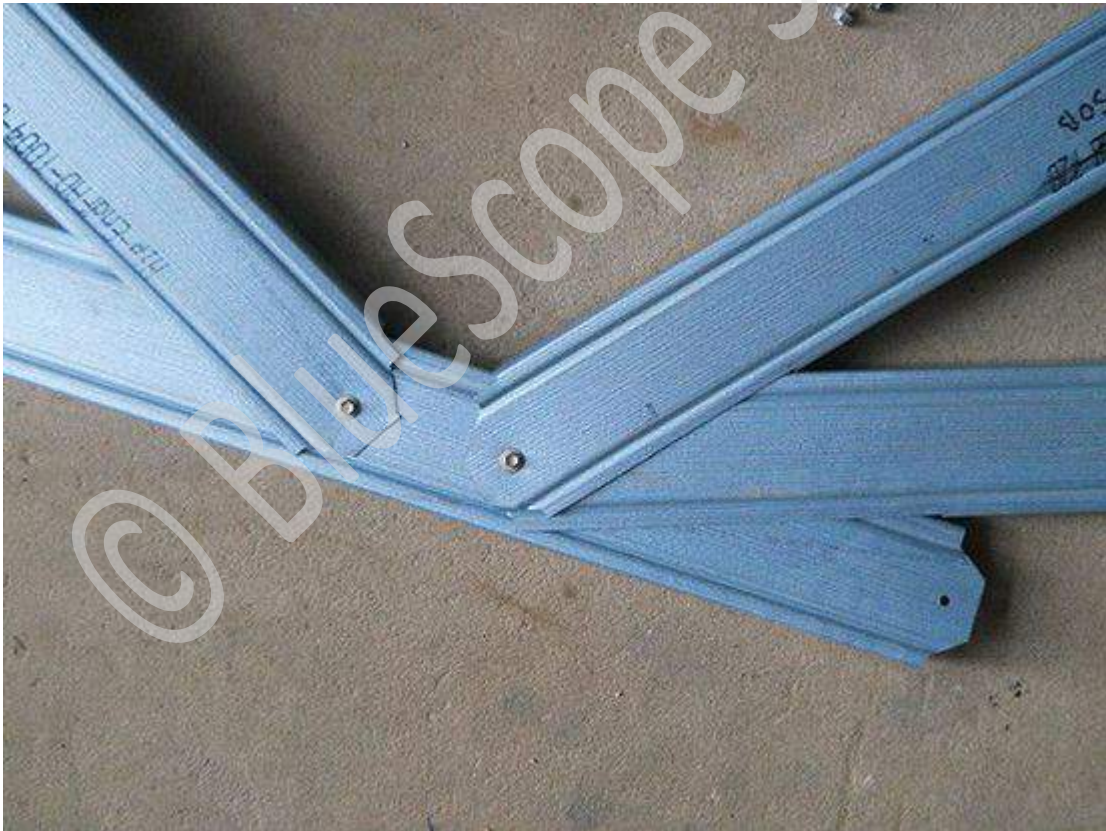
Finished connection (reinforced)
