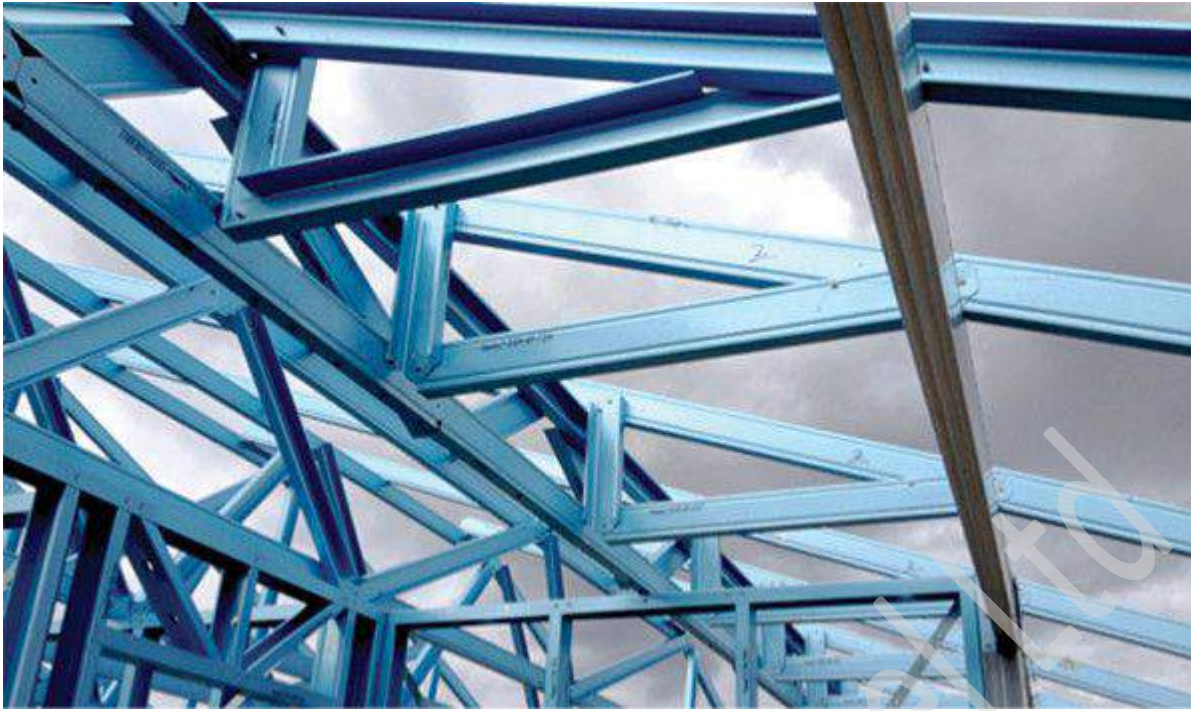
Figure 7.24a Installation of a Type 1A hip truss
