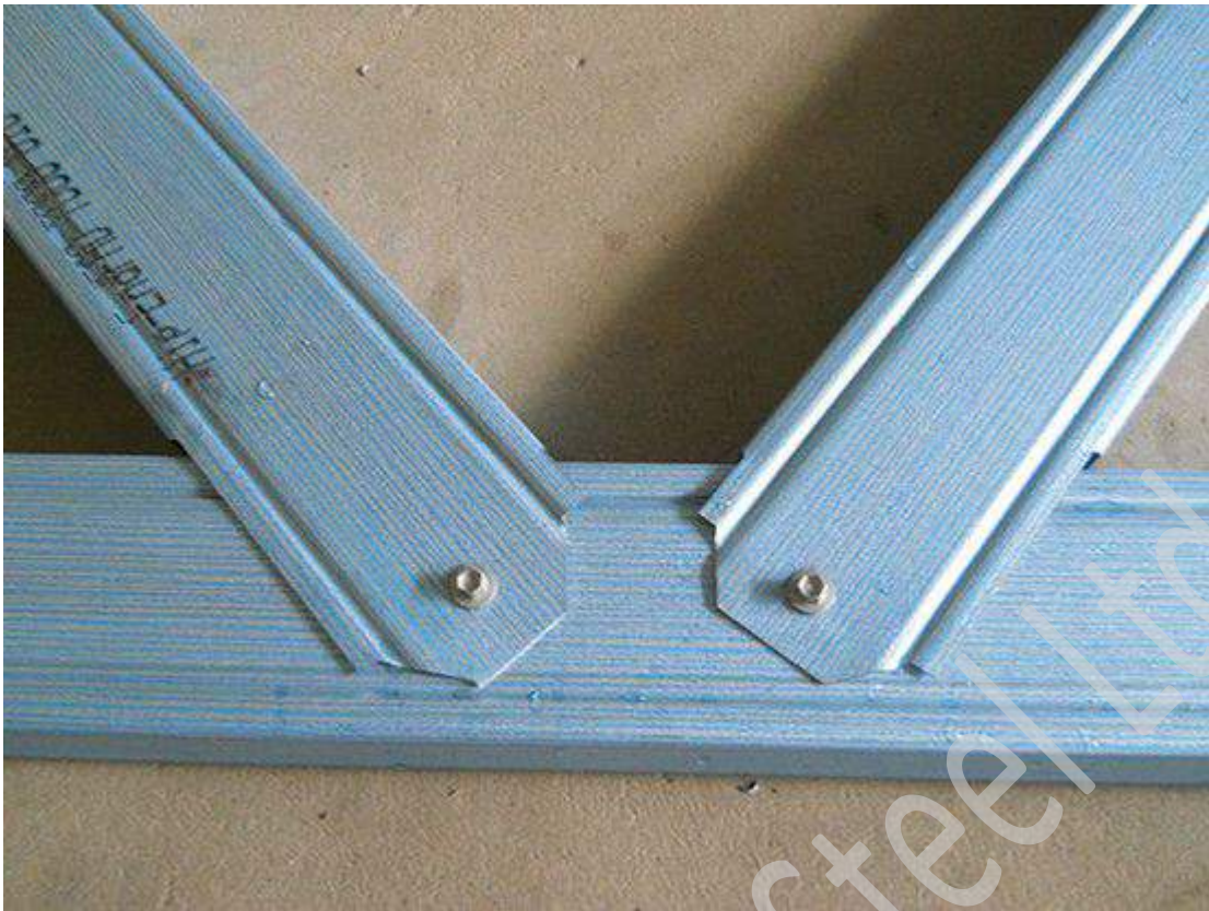
Finished knee web connection (unreinforced)
