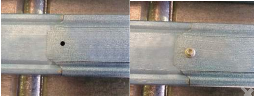
Figure 6.3 Bottom Chord connection at splice
