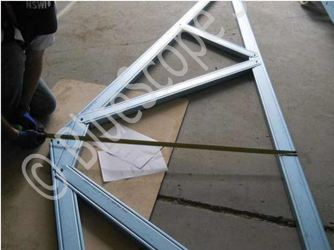
Finished connection (reinforced)
