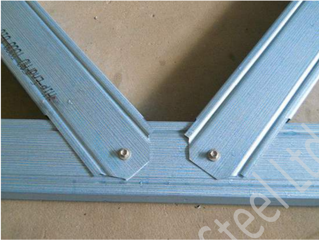
Finished knee web connection (unreinforced)
