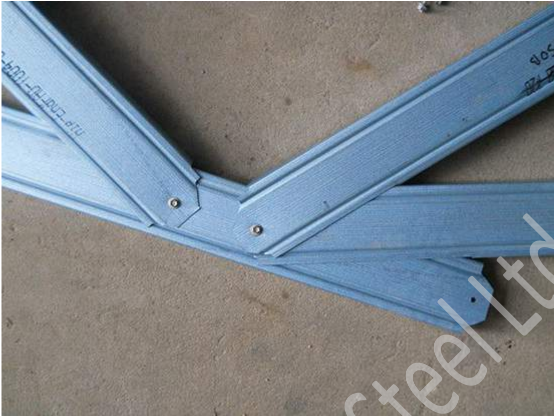
Finished connection (reinforced)
