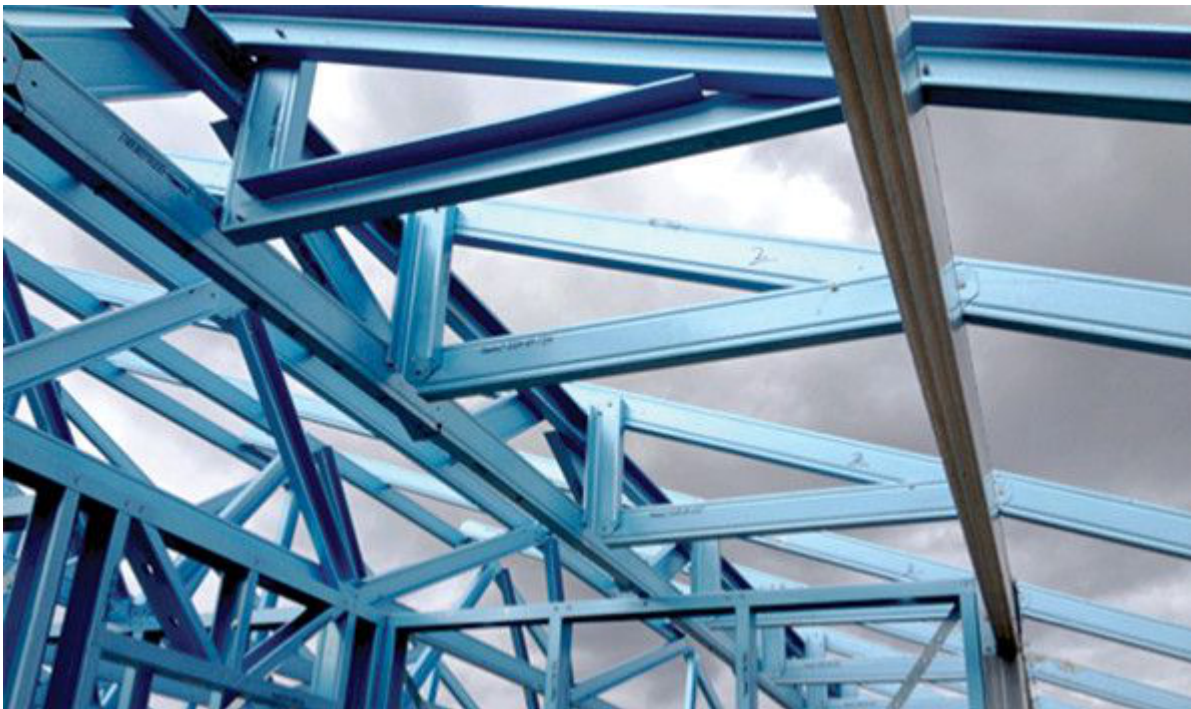
Figure 7.9 Installation of a Type 1A hip truss
