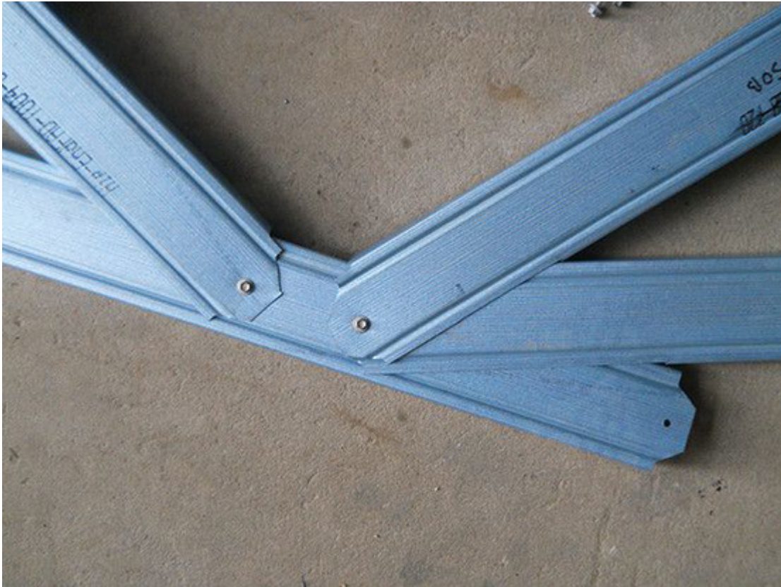
Finished connection (reinforced)
