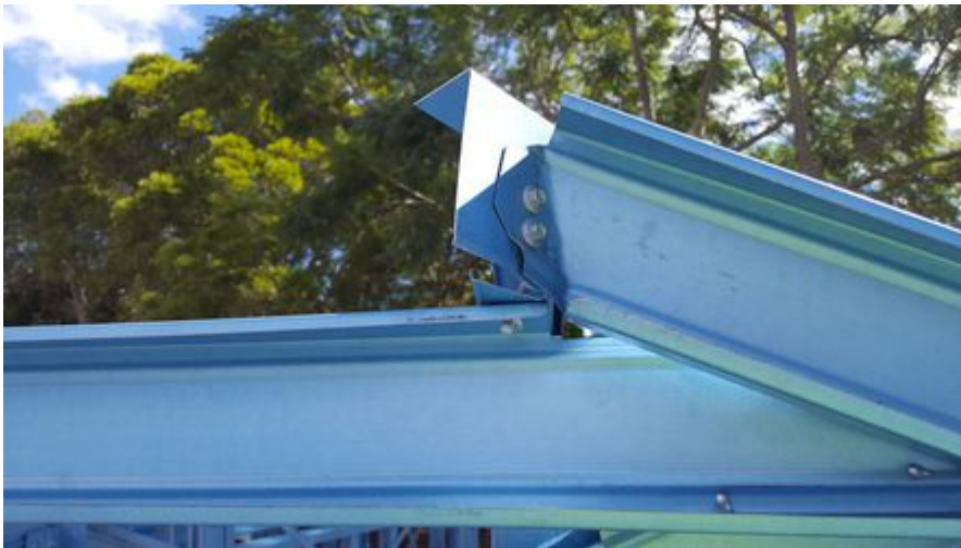
Figure 7.35 Veed hip rafter connecting to first station truncated truss (note: bottom flange of veed hip plate notched)
