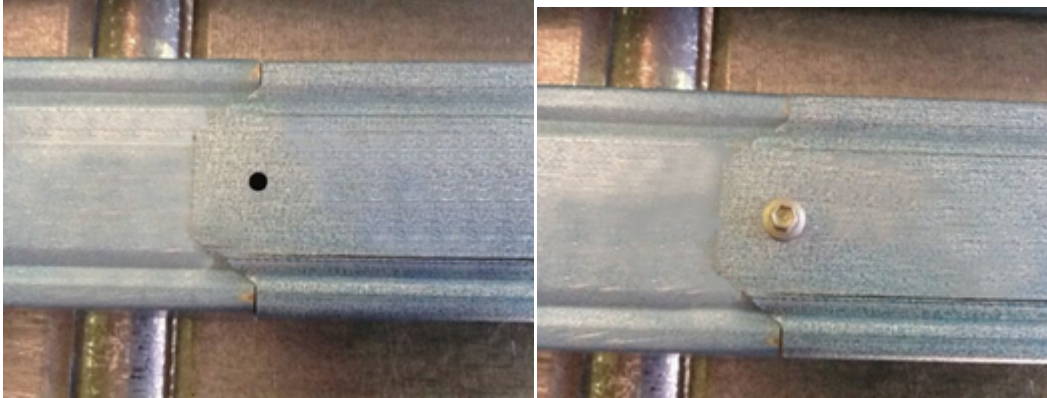
Figure 6.3 Bottom Chord connection at splice
