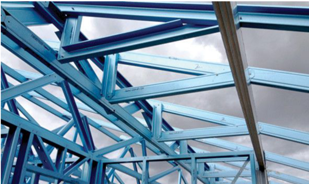
Figure 7.9 Installation of a Type 1A hip truss
