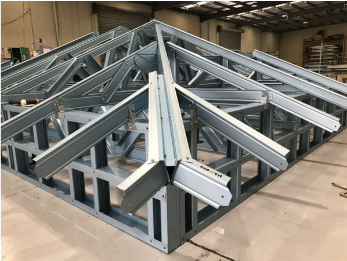
Figure 7.31: Veed hip rafters sitting on walls
