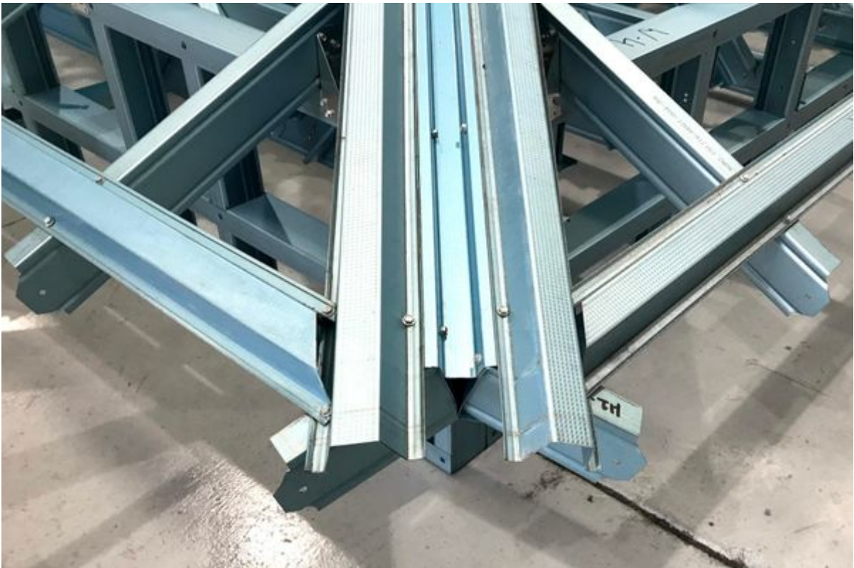
Figure 7.112: Veed hip rafter batten arrangement
