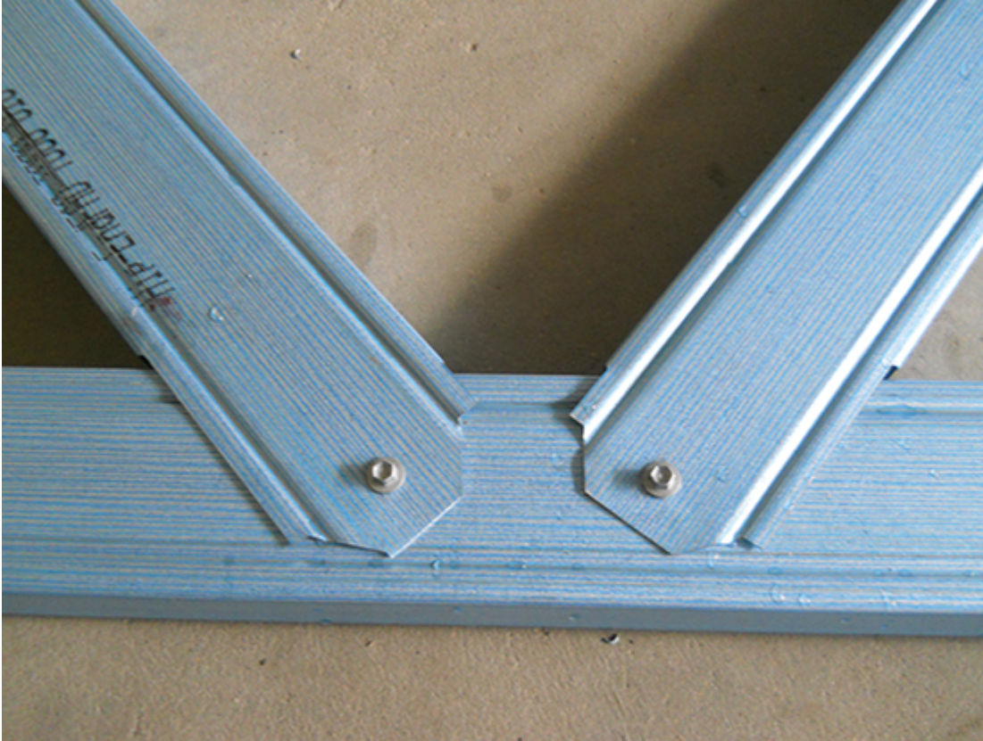
Finished knee web connection (unreinforced)
