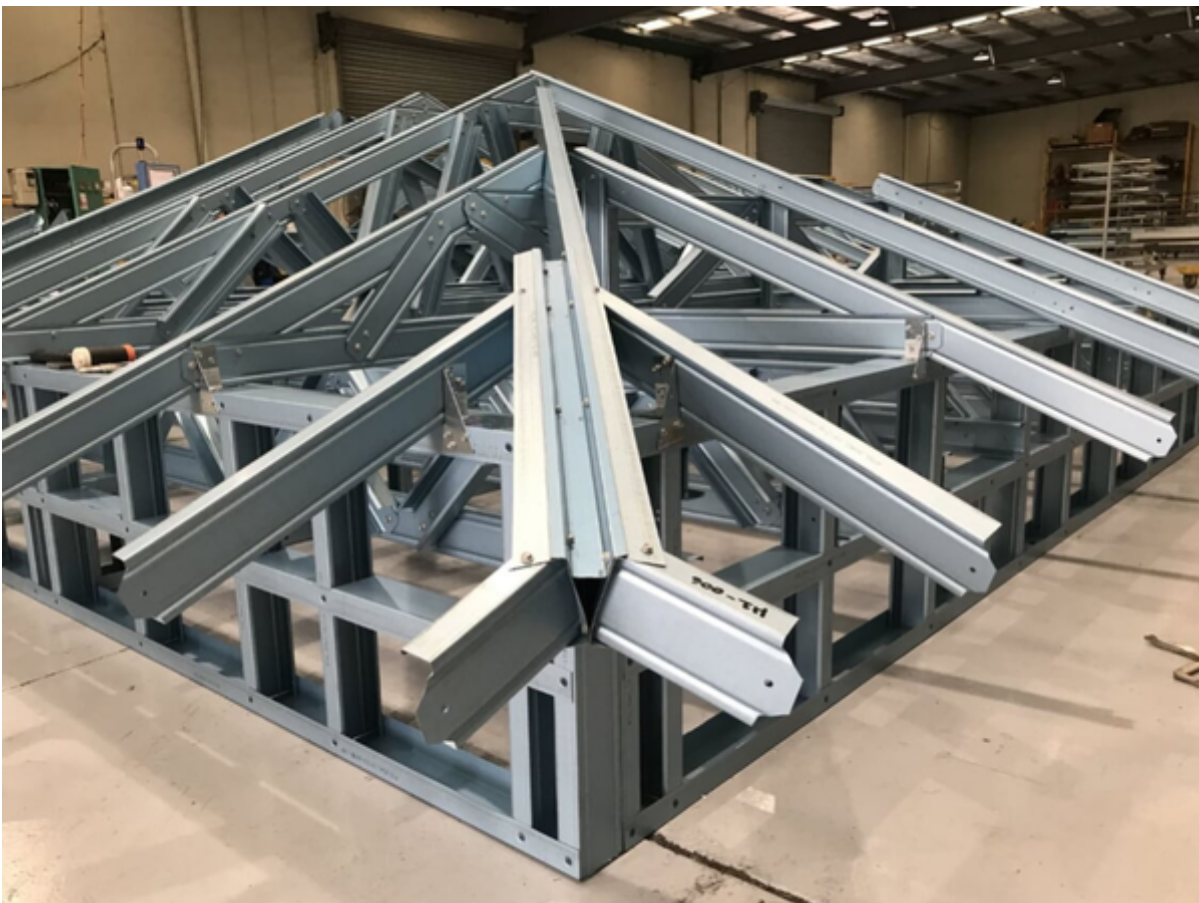
Figure 7.31: Veed hip rafters sitting on walls
