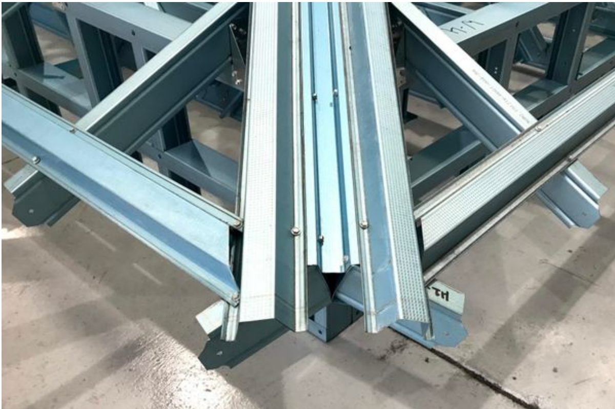
Figure 7.112: Veed hip rafter batten arrangement
