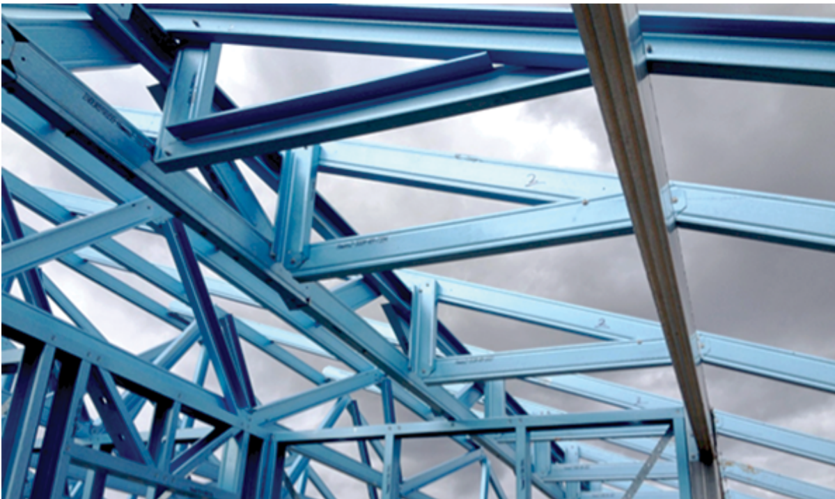
Figure 7.16: Installation of a Type 1A hip truss
