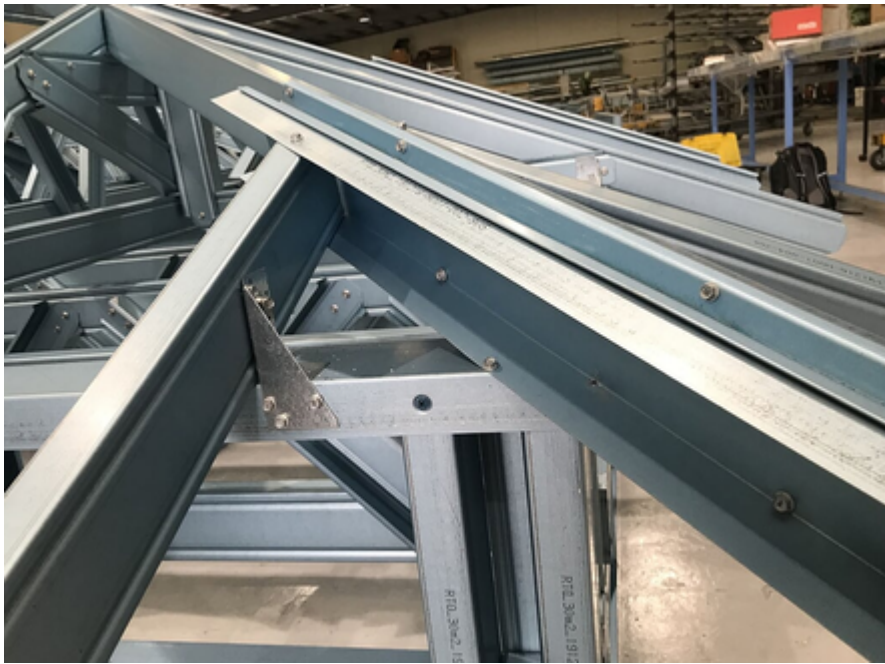
Figure 7.39 Fixing Veed Hip rafter to top plate
