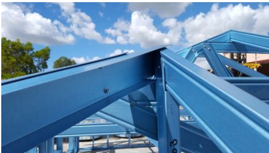
Figure 7.38 Veed hip rafter connecting to first station truncated truss (note: bottom flange of veed hip plate notched)
