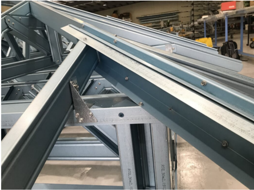
Figure 7.39 Fixing Veed Hip rafter to top plate
