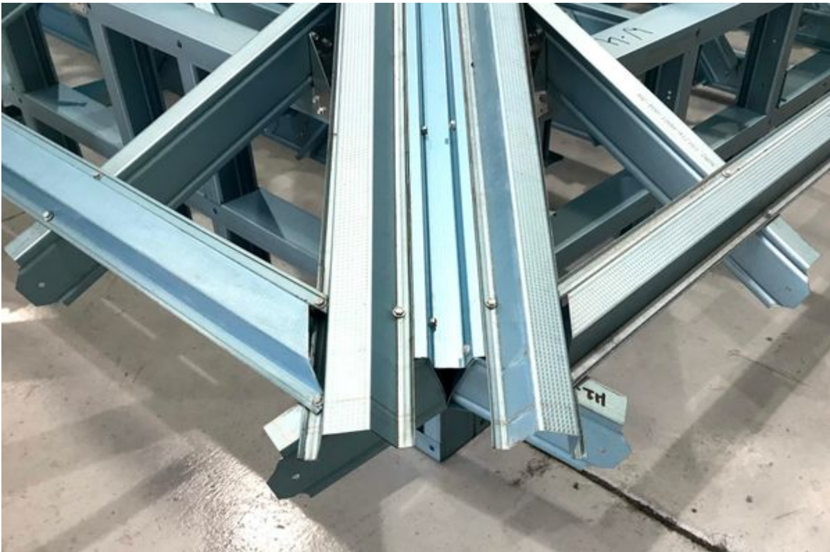
Figure 7.112: Veed hip rafter batten arrangement
