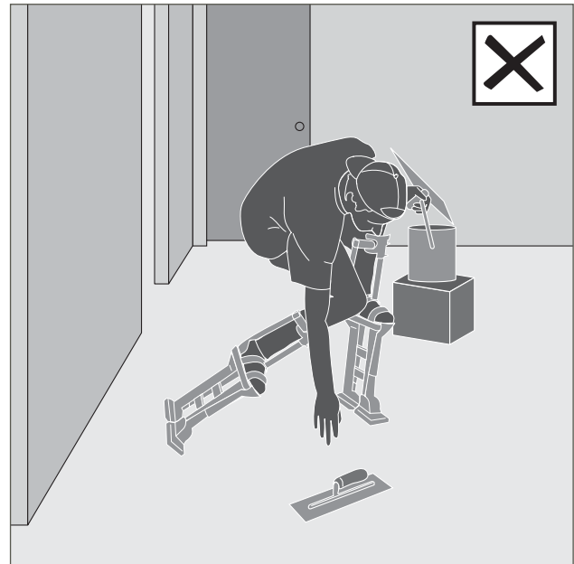
Figure 25 Inappropriate activity whilst on stilts – reaching below foot level stresses the knee, ankle, back and stilts.
