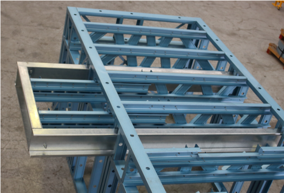
Detail: Example of cantilever truss end supported by beams which back span across floor
