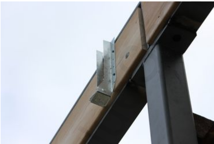
Detail: Locating joist hanger support brackets
