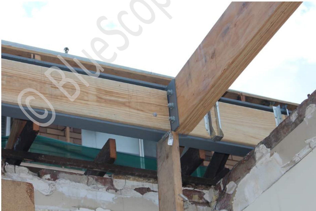
Picture: Fixing Secondary support beams
