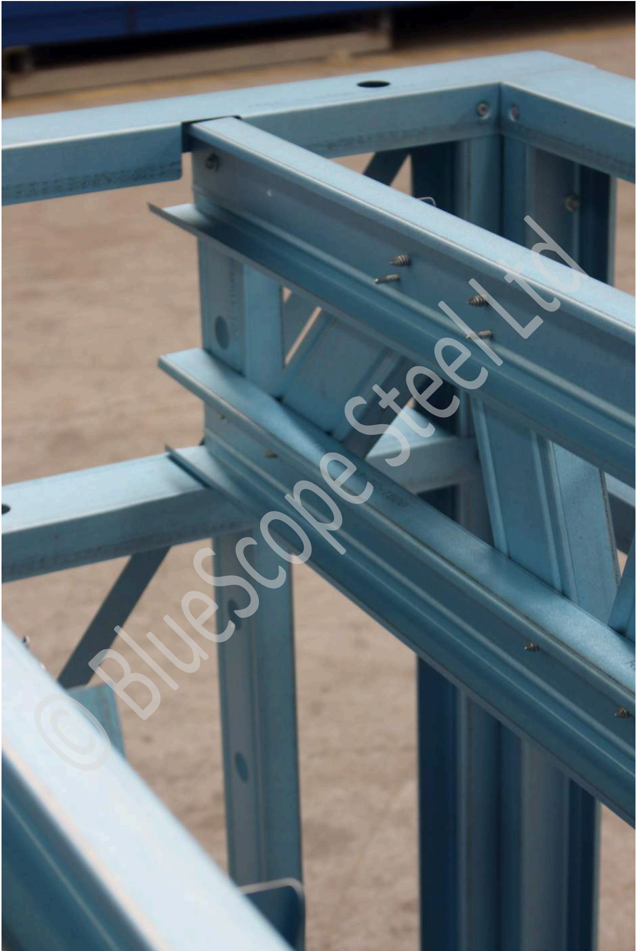
Step 8: Fix floor trusses to side of extended wall studs at the pre-punched hole location with 1 x Trusstite® per hole.
