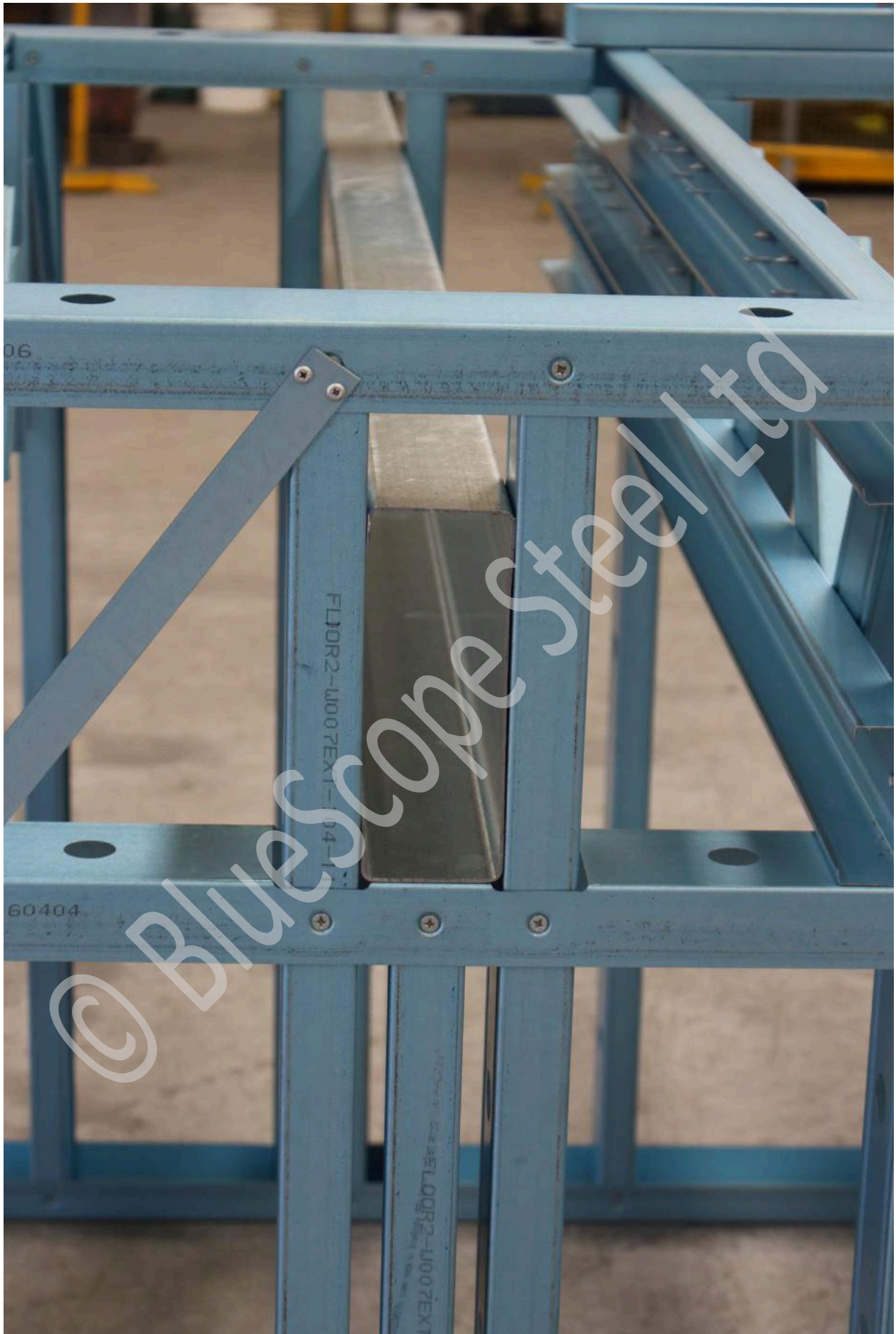
Step 5: Install connection brackets to secondary support trimming beams for floor trusses (Note: Connection to be specified by
