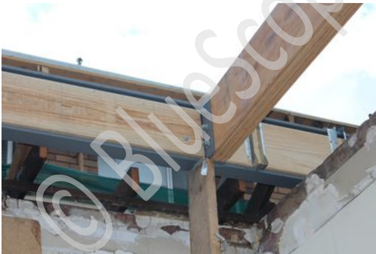
Picture: Fixing Secondary support beams
