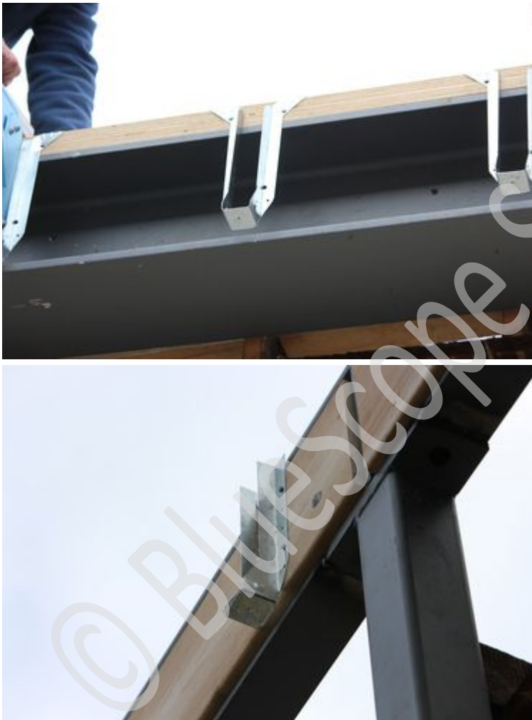
Detail: Locating joist hanger support brackets
