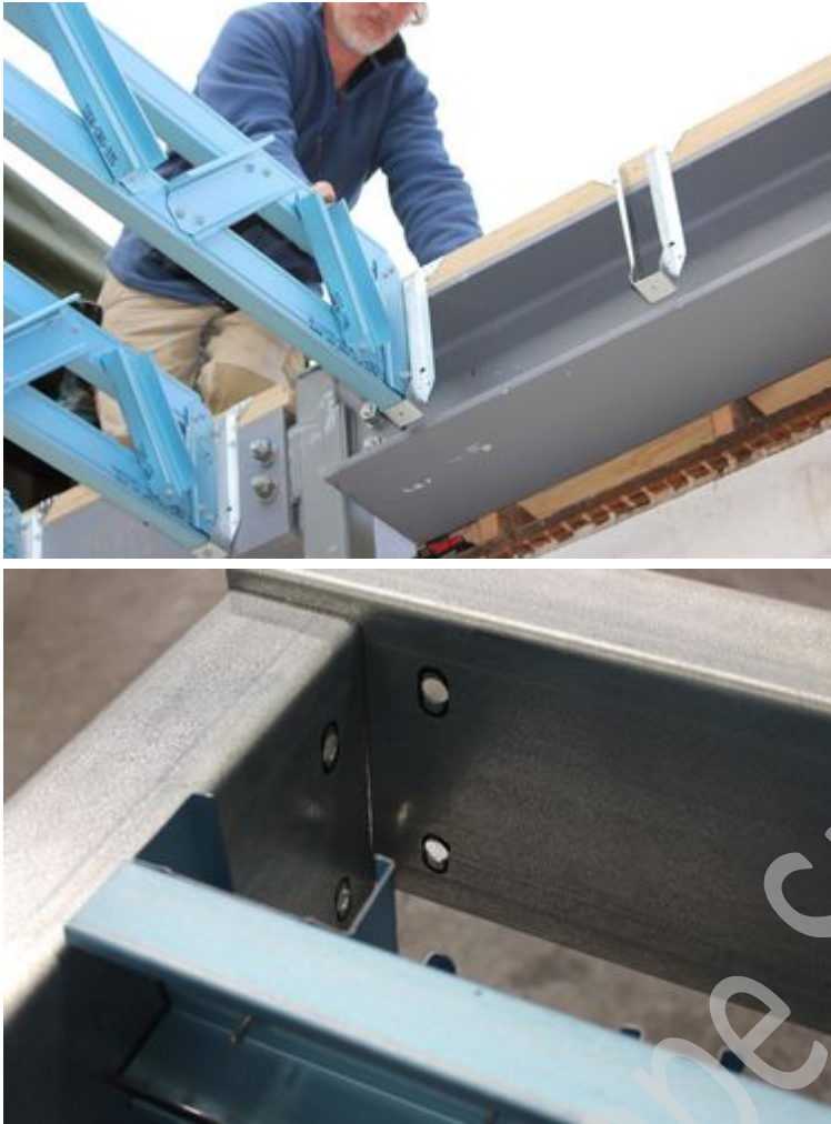
Picture: Packing beams
