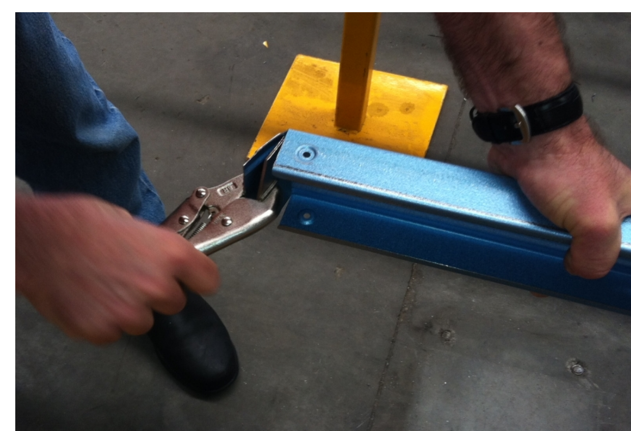
BEND BENT TAB WITH DUCKBILL PLIERS BEFORE FITTING IN FRAME
